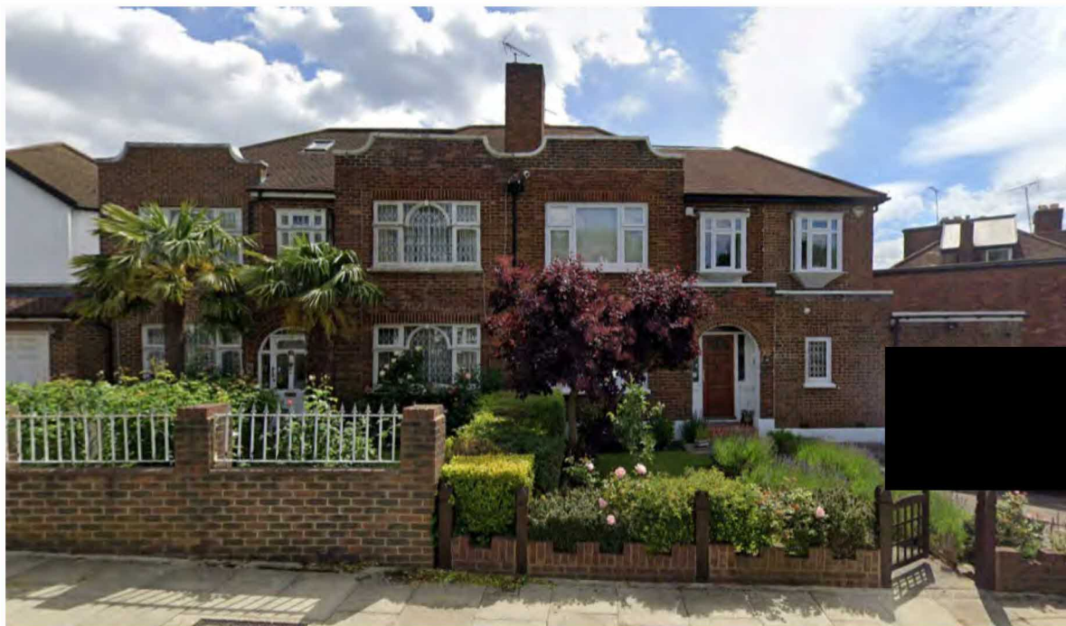
Existing front elevation - the mismatch of the ridge line between no 46 and 48 (left) is evident.
