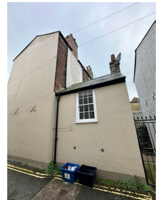
Existing rear extension. Added previous under planning application ref: 16/01350.
