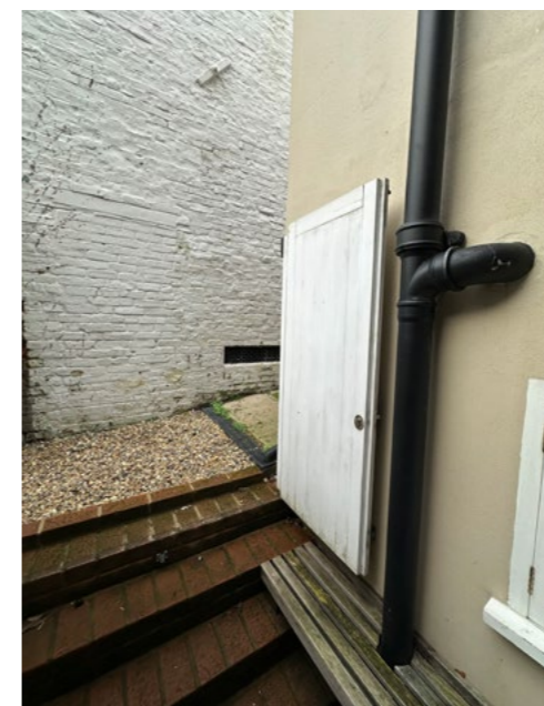
View towards alley from rear doorway.
