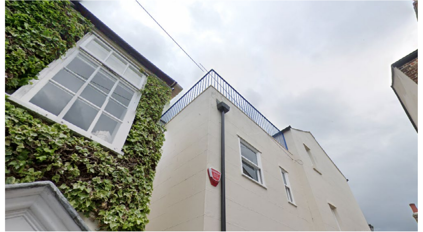
D House situated next door to our site - showing a rear terrace area & balustrade. Image courtesy of Google Maps
