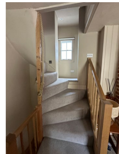
View from living room looking toward existing window that is proposed to become doorway.
