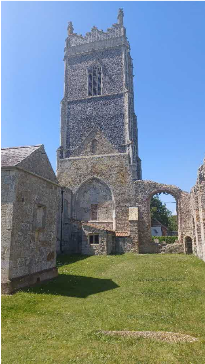
Figure 25 Image from within ruins of church looking west
