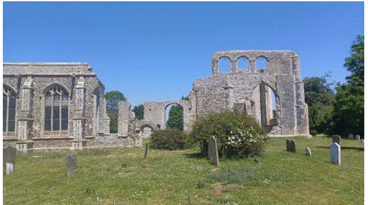
Figure 26 The ruined part of the church, from The Street
