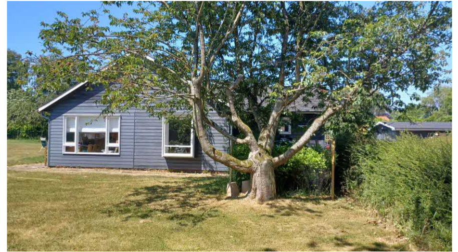
Figure 11 Side elevation, northeast
