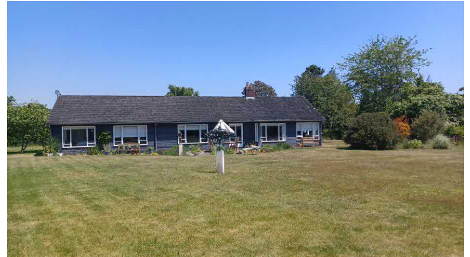
Figure 12 Rear elevation, south side
