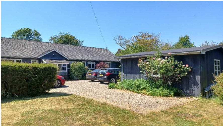
Figure 14 Side and rear of garage, northeast side, with house adjacent
