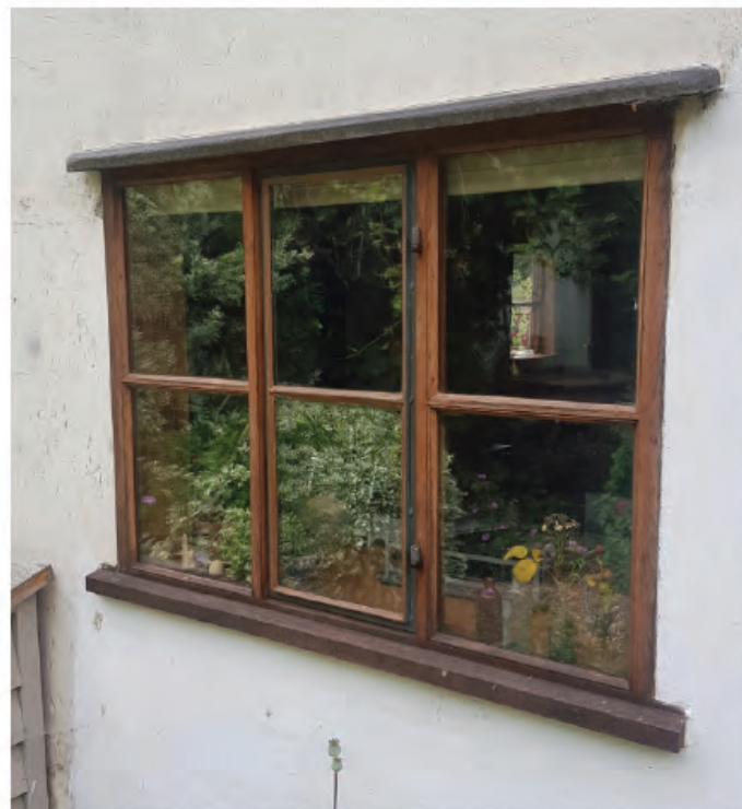
Pic. 32 Replacement windows.
