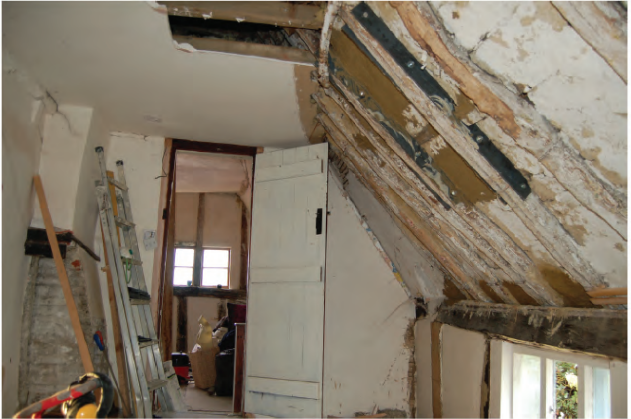
Plc 22 Bedroom 3 with roof rafters repaired using 10mm steel fitch plates
