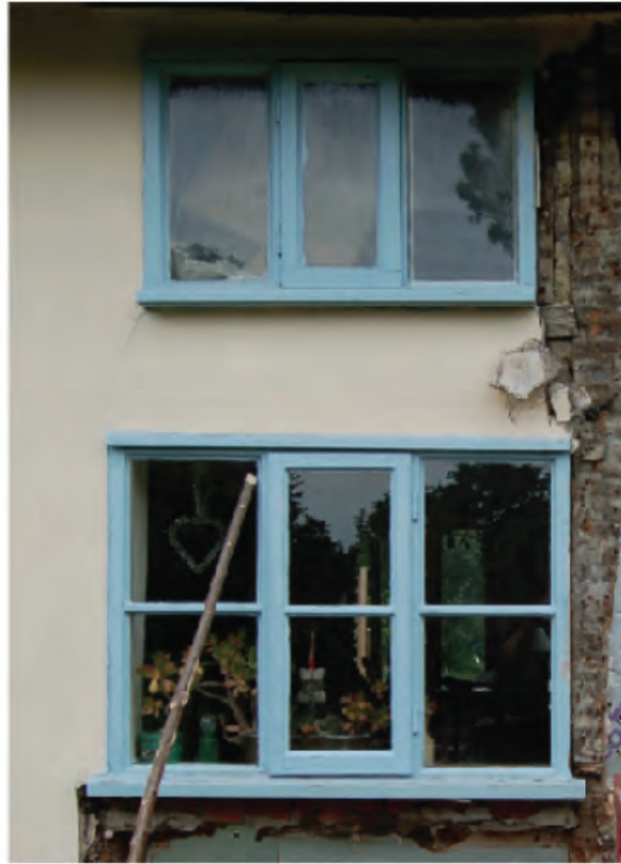
Pic. 31 Existing windows
