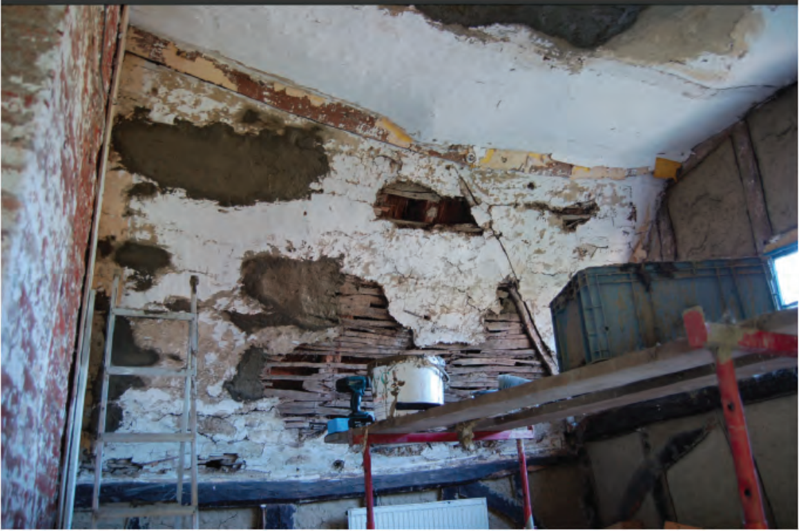
Repair to lath and earth plaster ceiling.
