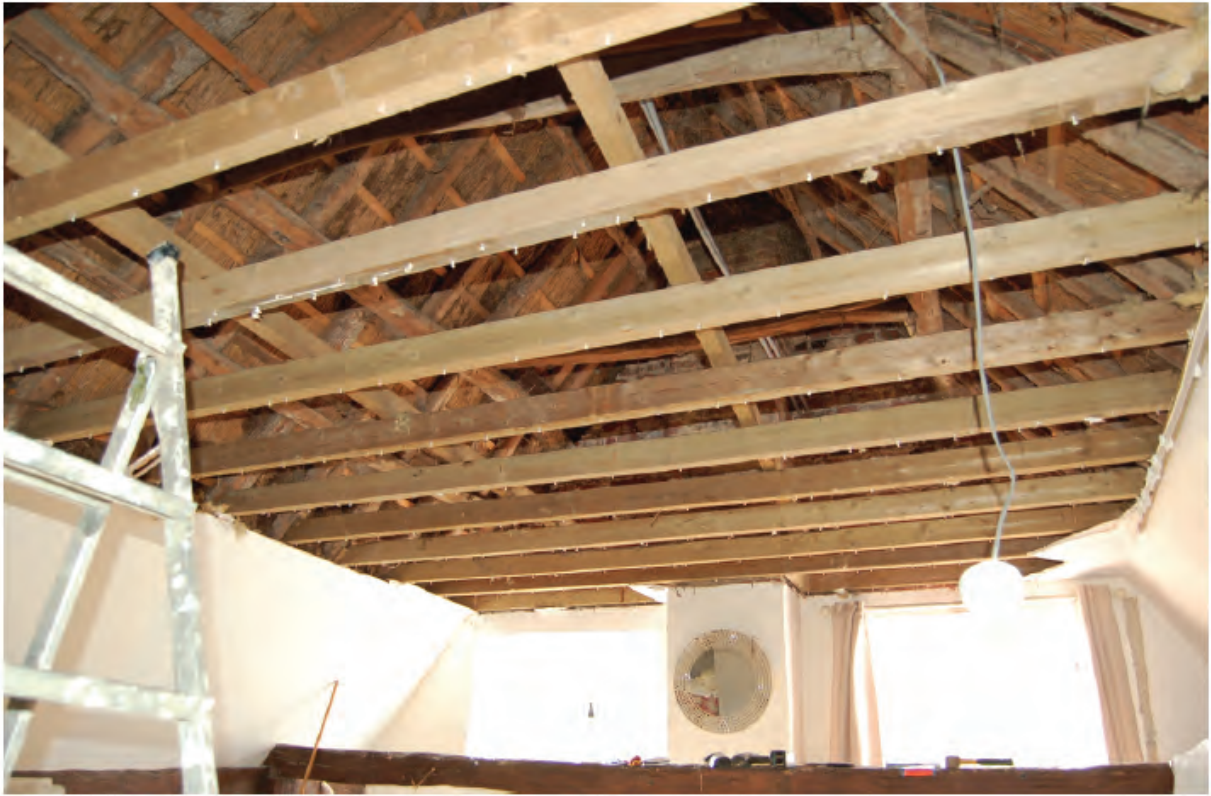
Removal of plasterboard ceiling
