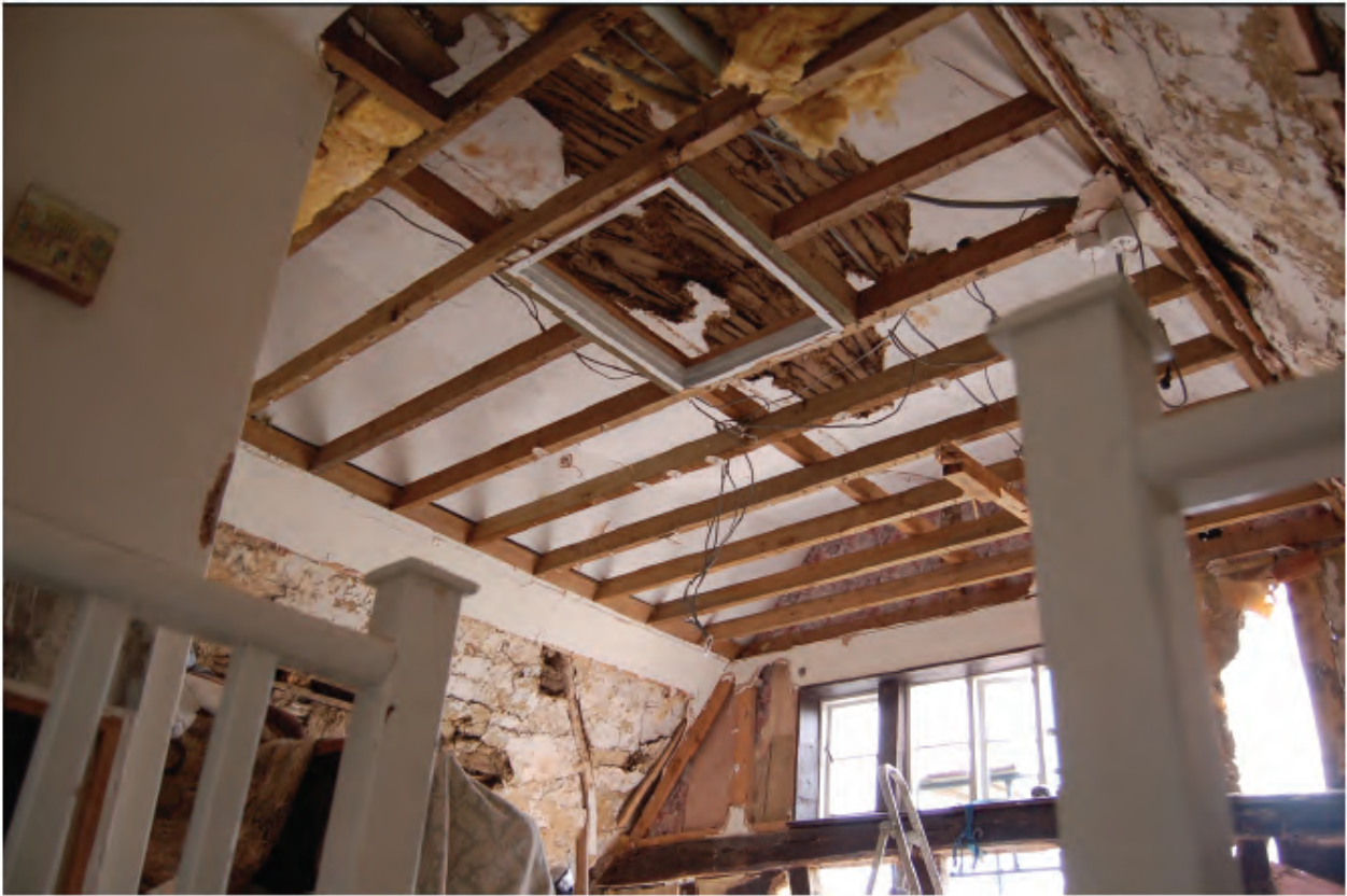
Plc 9 Removal of plasterboard ceiling.
