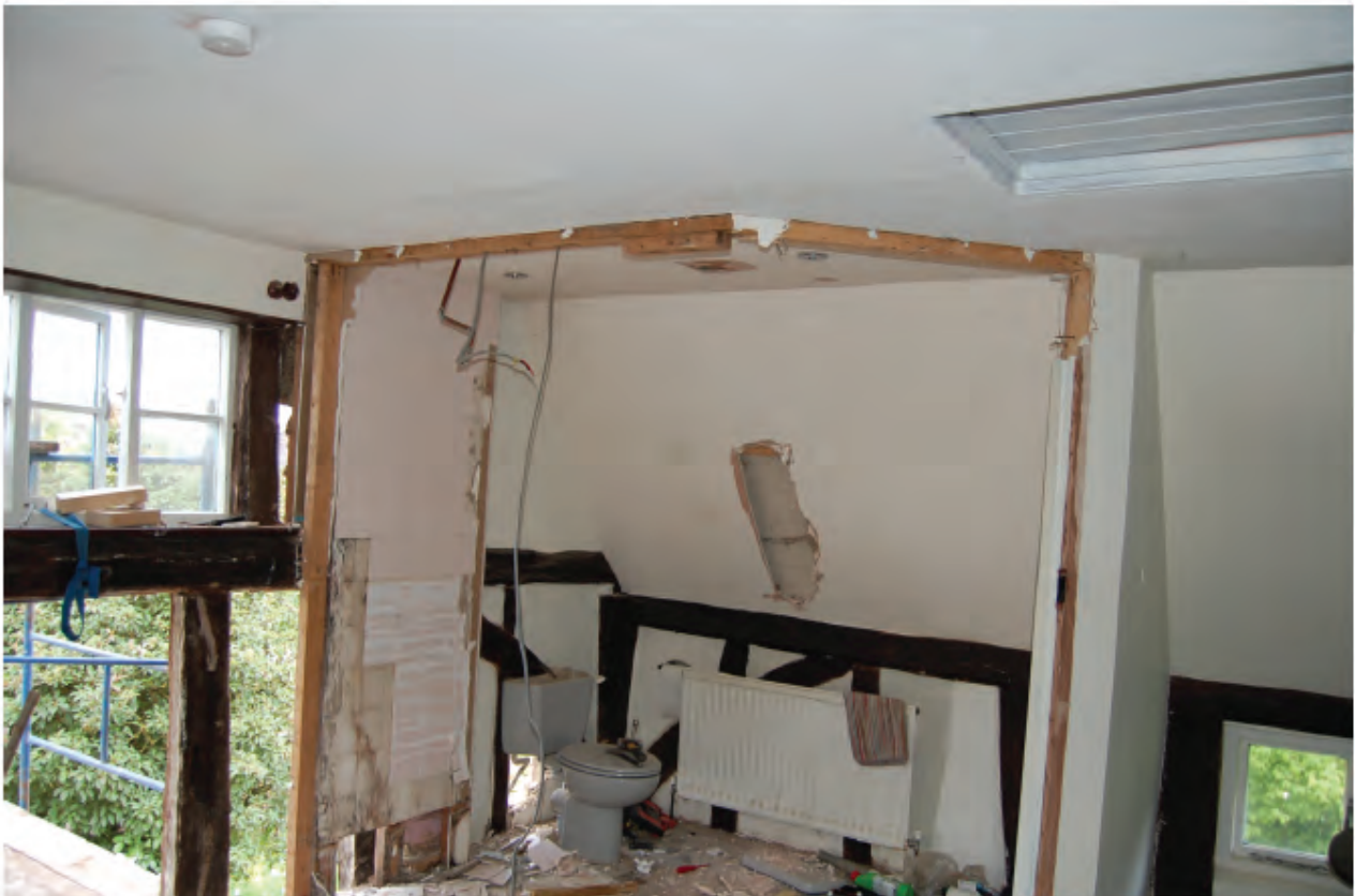
Plc 10 Removal of toilet and shower & plasterboard division in room.
