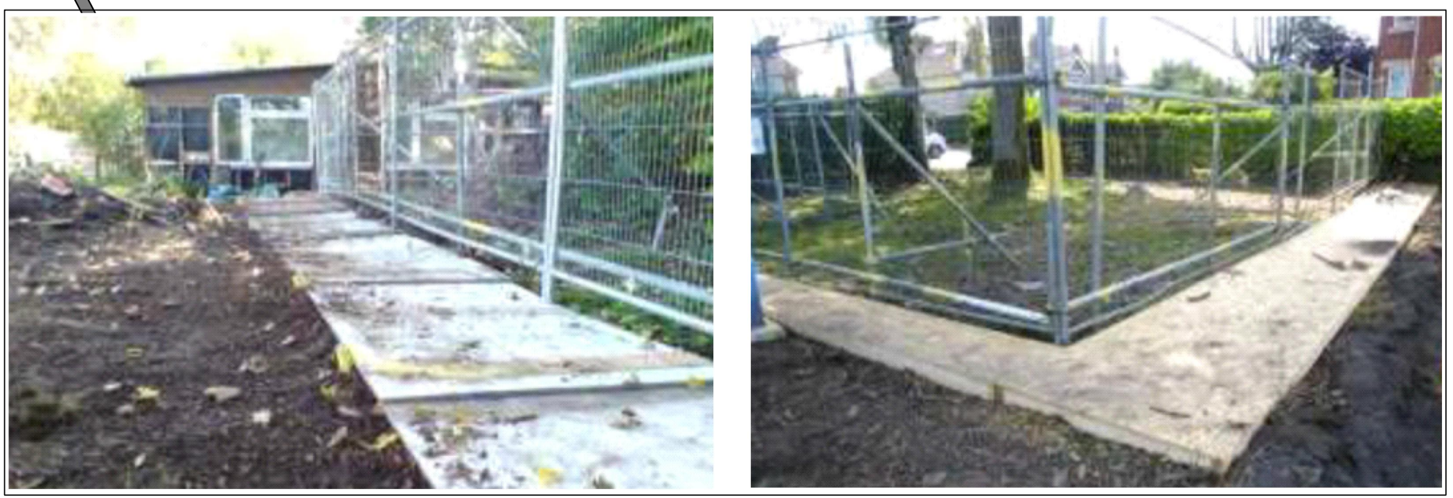
Examples of temporary ground protection suitable for pedestrian movements only - heavy-duty plywood sheets pinned into position (left) and plywood sheets fixed to a timber framework (right)
