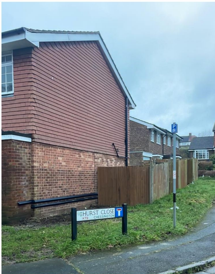
PHOTOGRAPH – Original fencing
