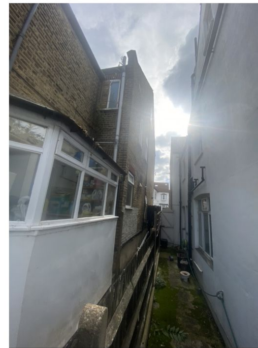
Photo showing side passageway
