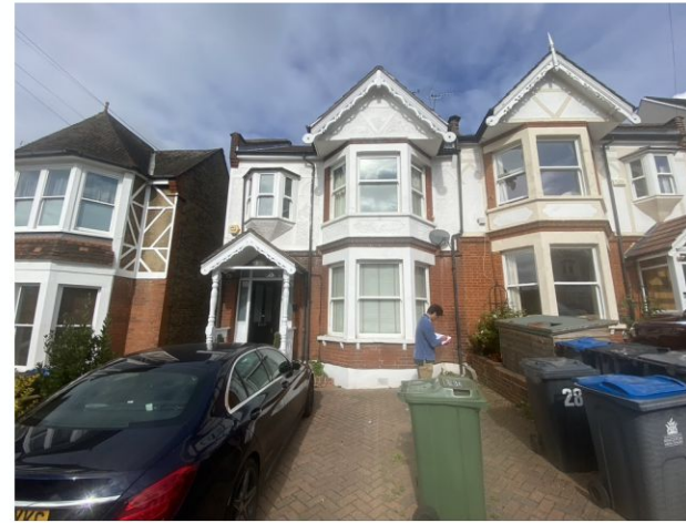
Photo showing front elevation from Dukes Av.
