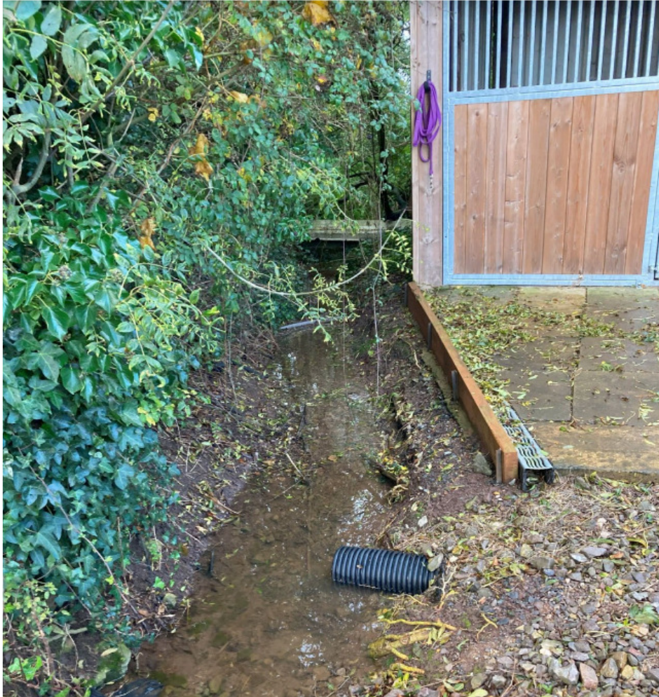
Photo 1: Outfall from site to culvert across Field Lane
