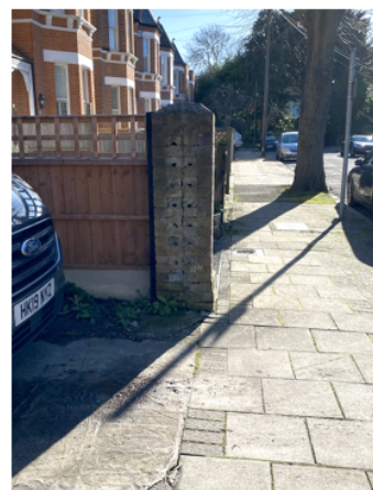
Righthand side. 1.2m high pier to neighbouring boundary - can't be moved
