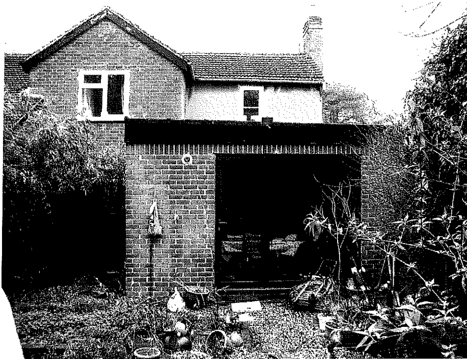
P.2. Rear Elevation (including the gable end of No.14 Queen Street)
