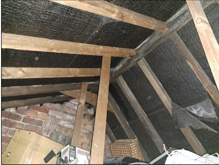
Photograph 6: Showing roof lining.
