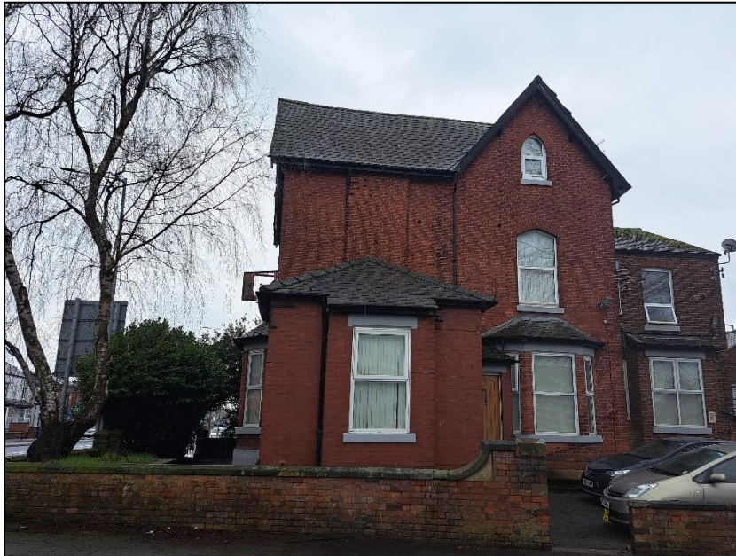
Photograph 1: Showing exterior to the north.
