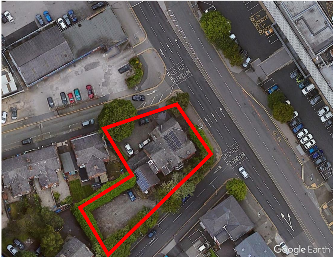
Site plan indicating the extent of the site and the surrounding environment
