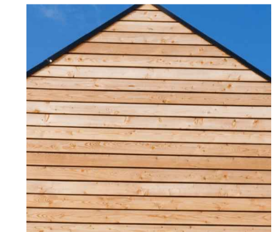
Timber cladding to gable end
