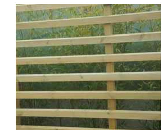
Hit & miss horizontal timber cladding
