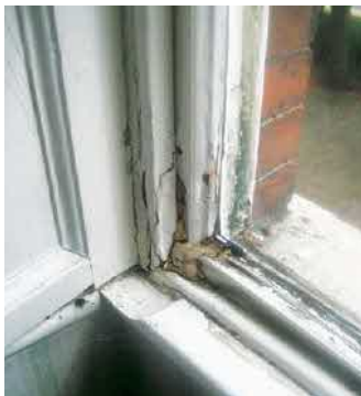
Above: Rotten and decayed windows like these are the typical Job Kierson is asked to help with. The fully restored windows (top right) in this Grade II* property contributed to Kierson's recent Civic Society Heritage Building Award
