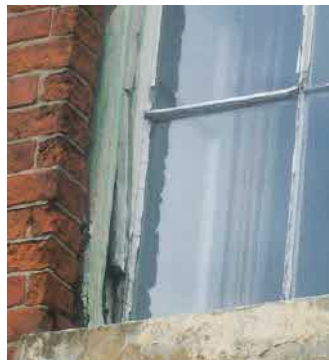
Above: Rotten and decayed windows like these are the typical Job Kierson is asked to help with. The fully restored windows (top right) in this Grade II* property contributed to Kierson's recent Civic Society Heritage Building Award
