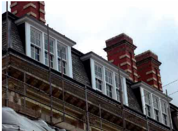
Dormer windows on part of the Railway Offices, Altrincham, part of a 400-window restoration
