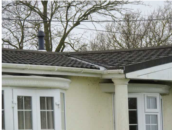
Photo 5: Showing tight seal to roof
