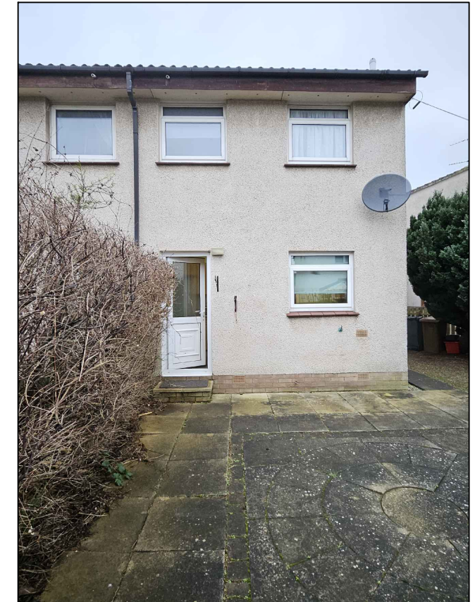
Existing Photo Rear Elevation
