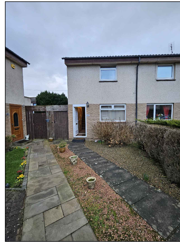
Existing Photo Front Elevation
