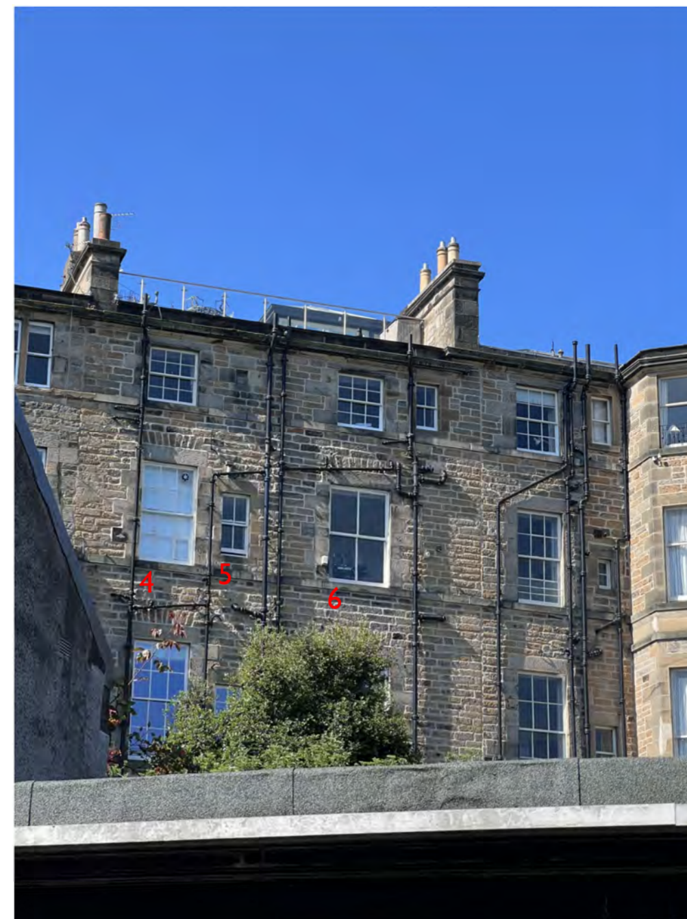
Photo of Rear Elevation
