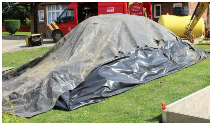
Figure 4.18.6 – Backfill covered with tarpaulin to be kept dry.
