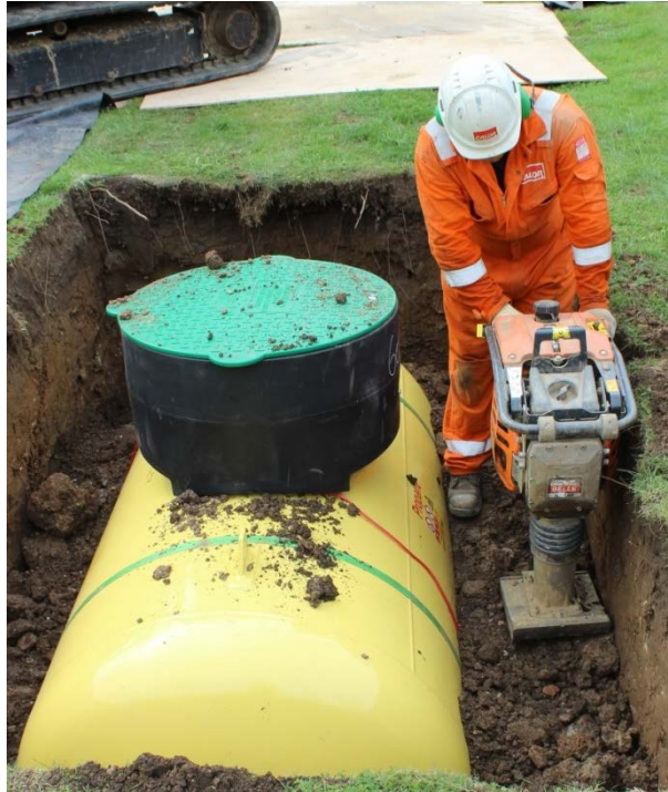
Figure 4.18.7 – Compacting the backfill using a vibro tamper
