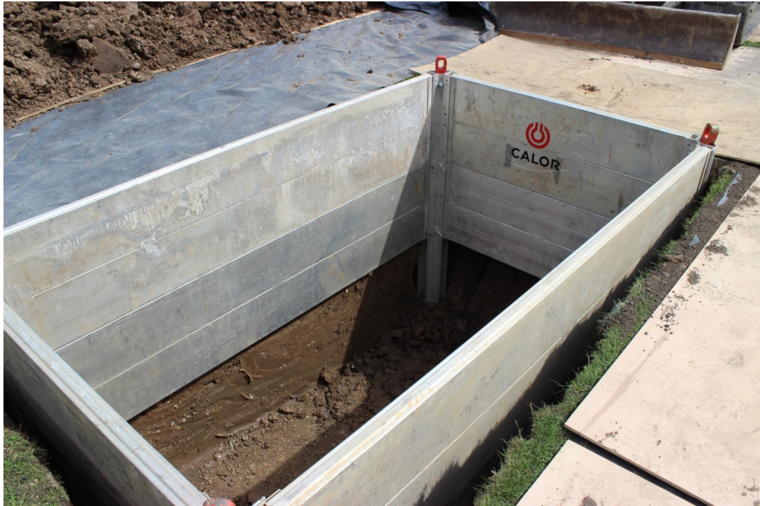
Figure 4.18.1 – Example of an excavation support system
