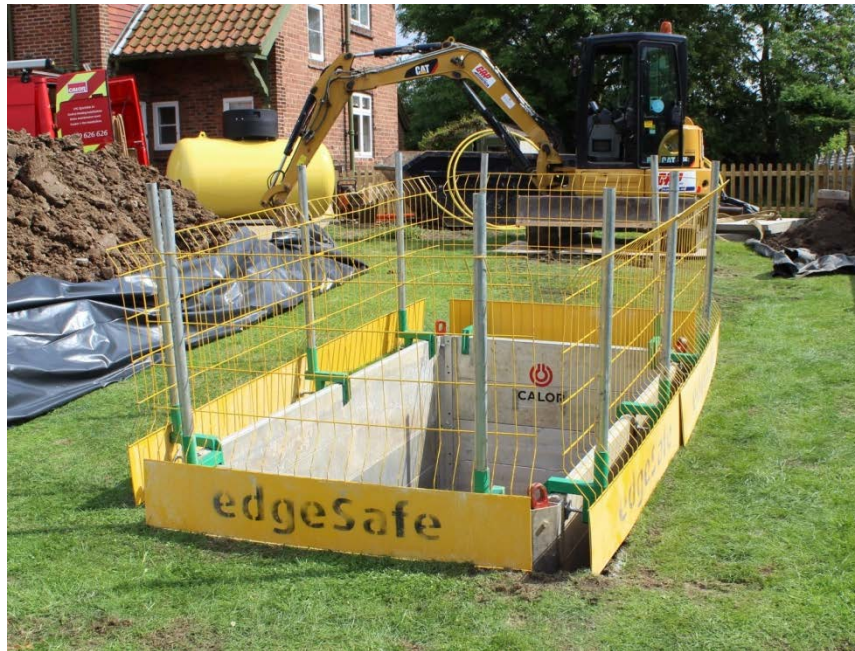
Figure 4.18.5 – Excavation with safety barrier
