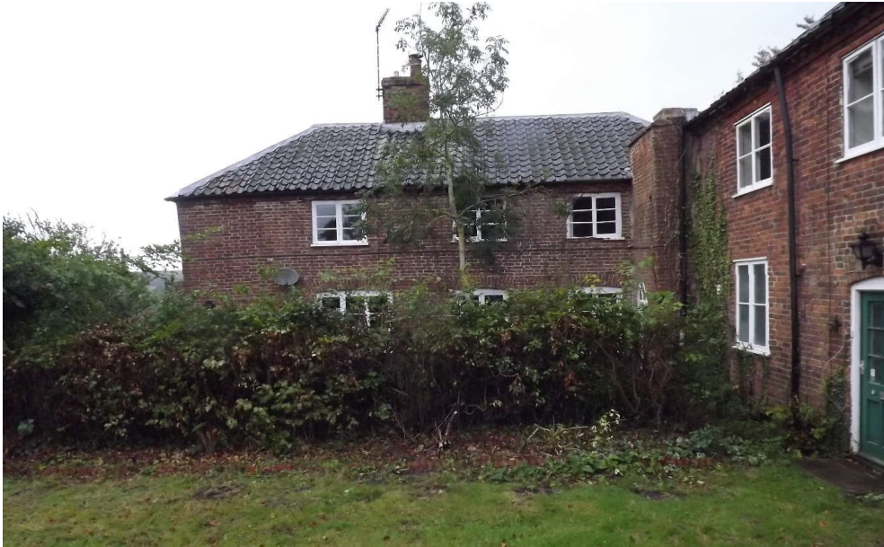
Existing 9 and 10 West Raynham Road
