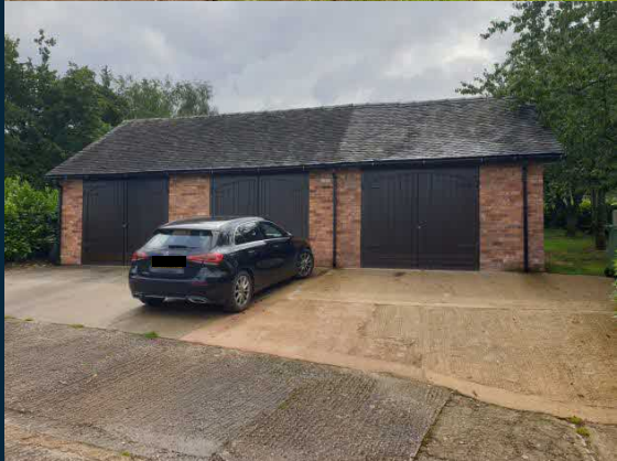
Subject garage front and rear elevations
