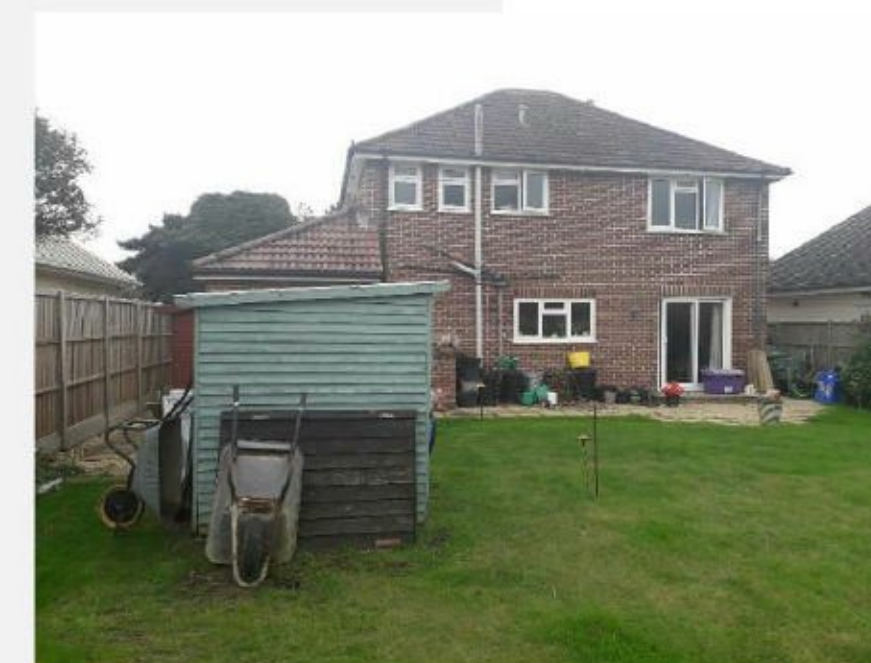
View towards rear of existing house
