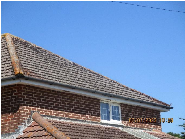
Photo 4: East elevation of house.
