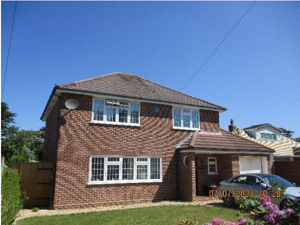
Photo 1: South elevation of house.
