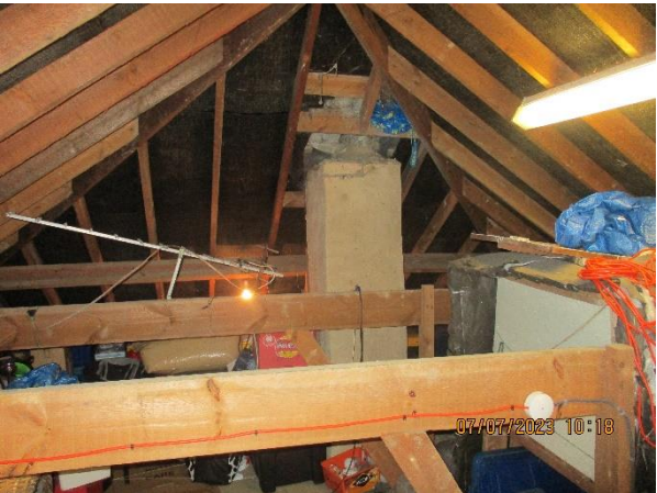
Photo 5: Internal loft void of house.
