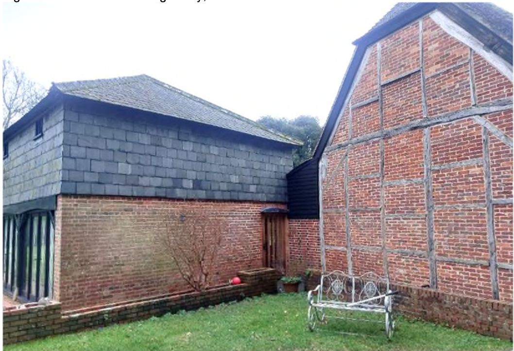
Figure 4 The west gable of the cart shed and granary with the north gable of the linked barn to the right.
