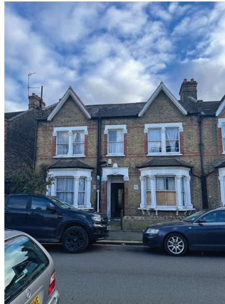
View of front elevation of 25 Surrey Road
