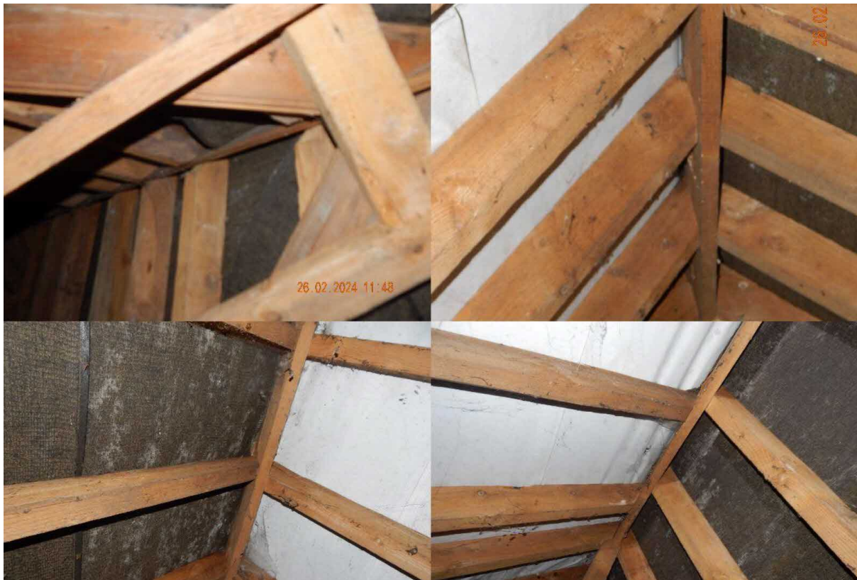
Image 10 – B1 – Evidence of felt/PVC membrane coverings below the tiled roof coverings
