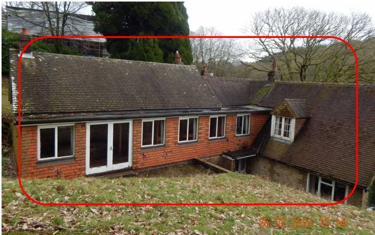
Image 8 – B1 – North & West facing elevation of the property offering further gaps of value to bats within the roof and vertical tile coverings
