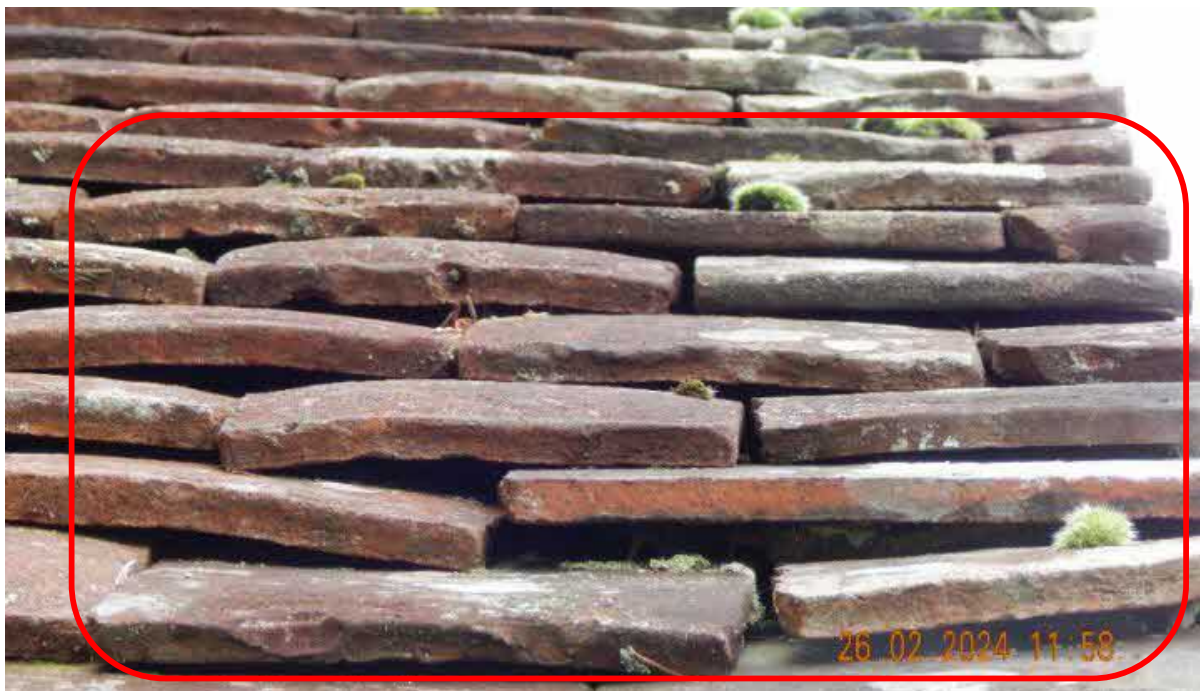
Image 5 – B1 – Further features of value to bats across the lower front roof coverings with likely roosting habitats within
