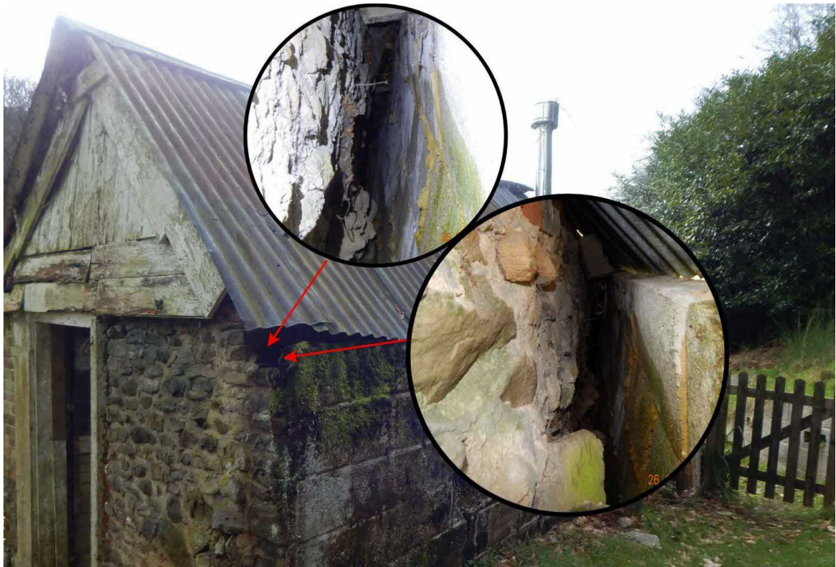
Image 13 – B2 – North elevation offering enclosed crevice spaces of value to bats
