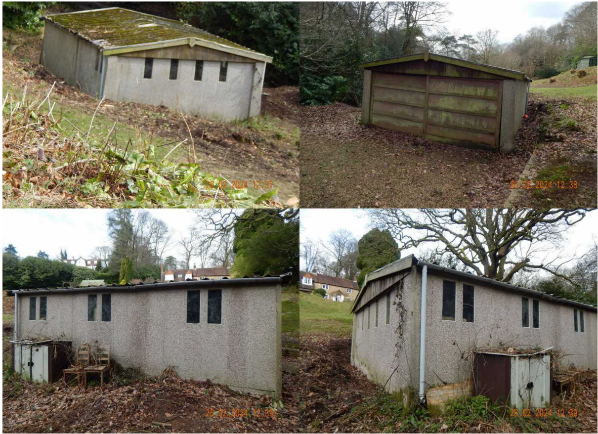
Image 17 – B4 – Fabricated garage structure
