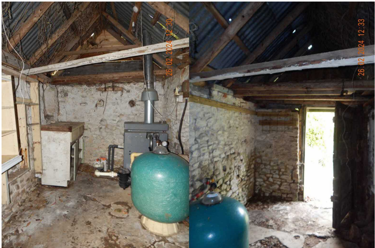
Image 14 – B2 – Internal view from within the structure
