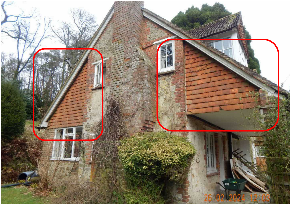
Image 6 – B1 – West facing elevation of the property where the proposed development works will take place. Further features of value to bats were observed within the vertical hanging tiles
