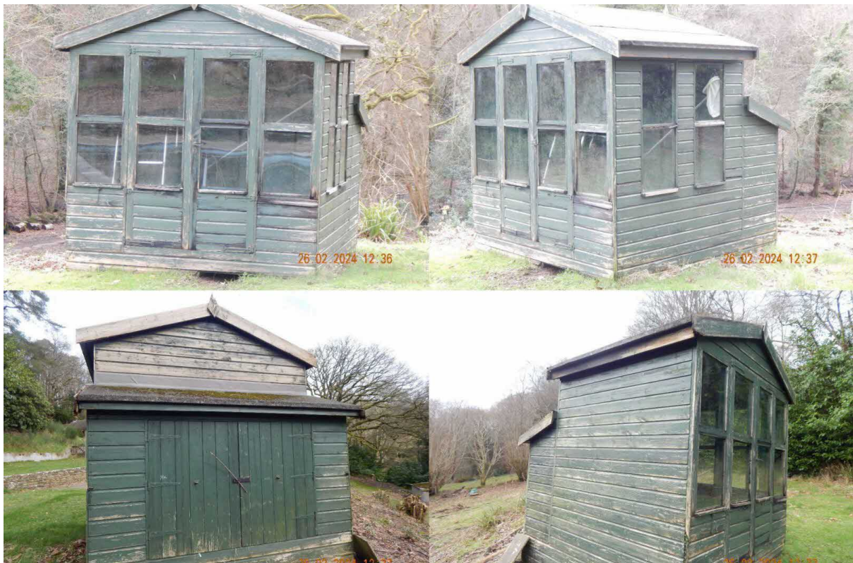
Image 16 – B3 – Timber fabricated structure
