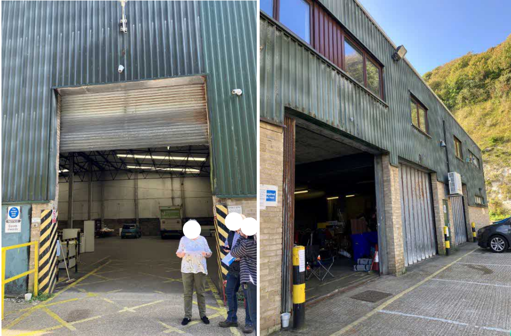
Figure 3-2: Existing warehouse access to be used as the car park entrance and exit points
