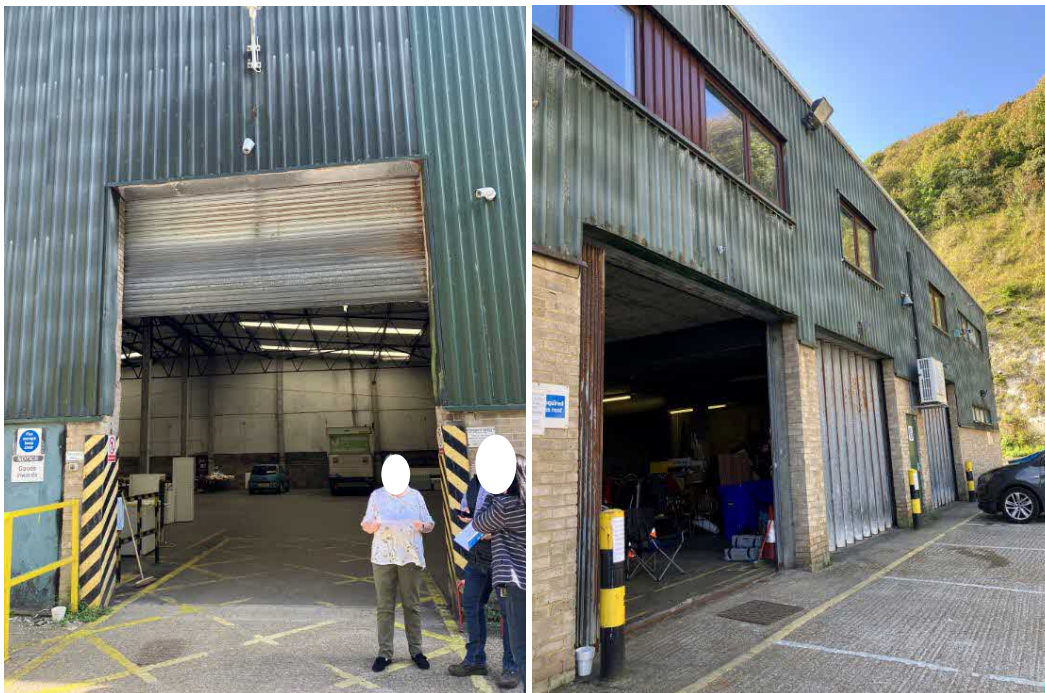
Figure 3-4: Existing warehouse access to be used as the car park entrance and exit points
