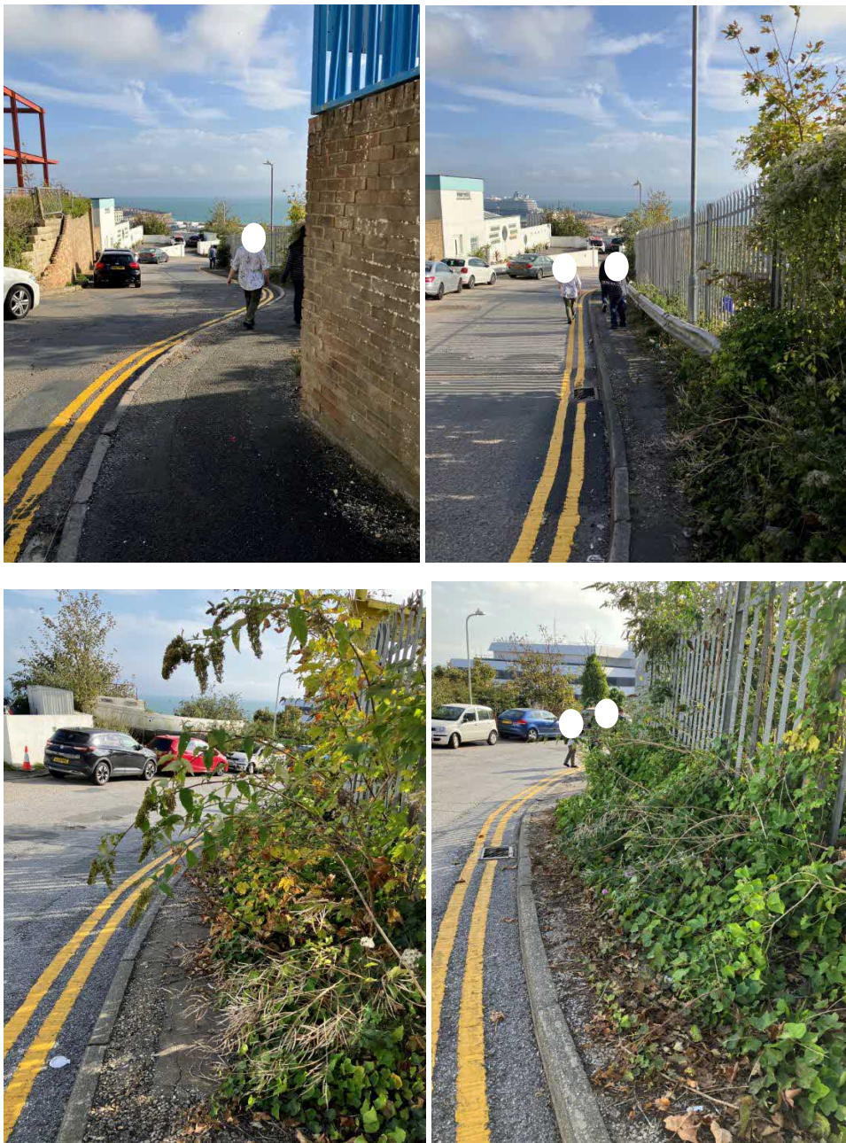
Figure 2-4: Pavement along Channel View Road
