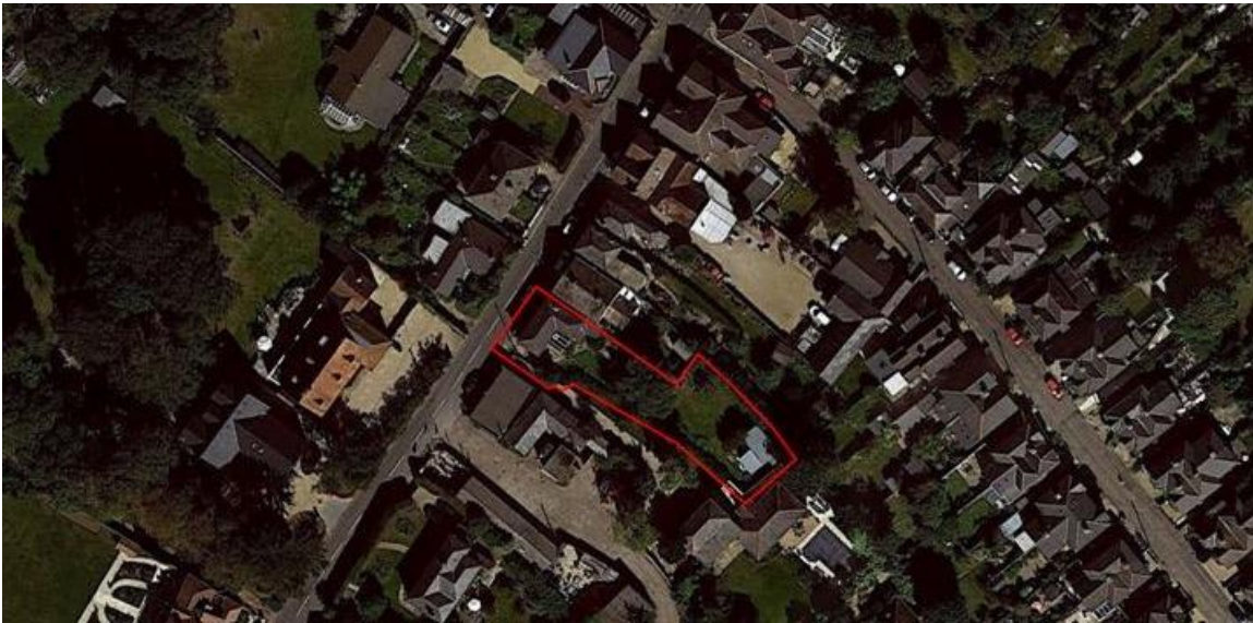
Aerial view of 69 High Street.
