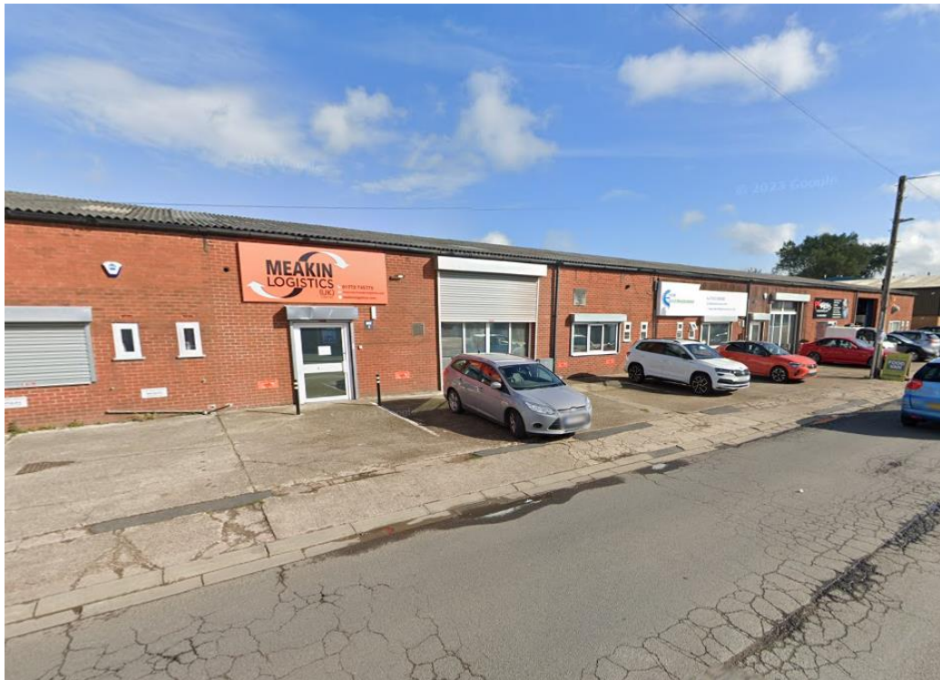
Above: Image above shows the front elevation of the building with its large glazed opening and shutter, separate pedestrian door, and parking area adjacent.
