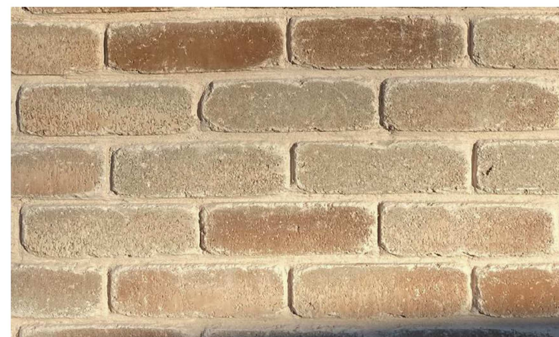
BRICK FINISH 02 - Brick with raked back mortar F10/215 1:10
