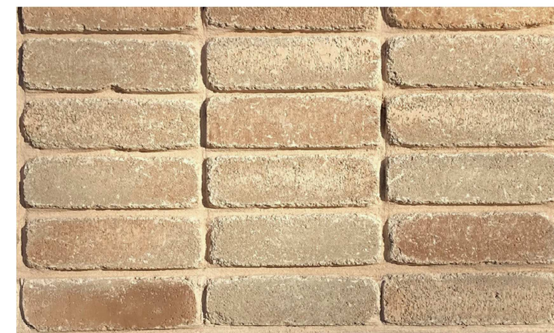
BRICK FINISH 03 - Stack bonded brick F10/215 1:10
