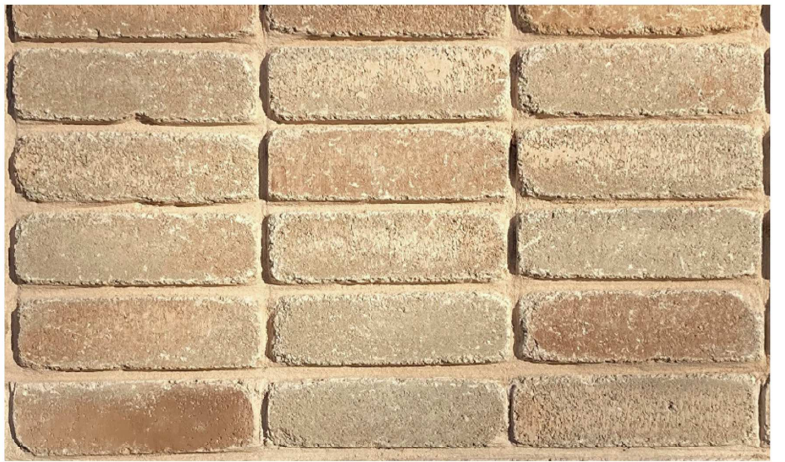
BRICK FINISH 03 - Stack bonded brick. F10/215 1:10
