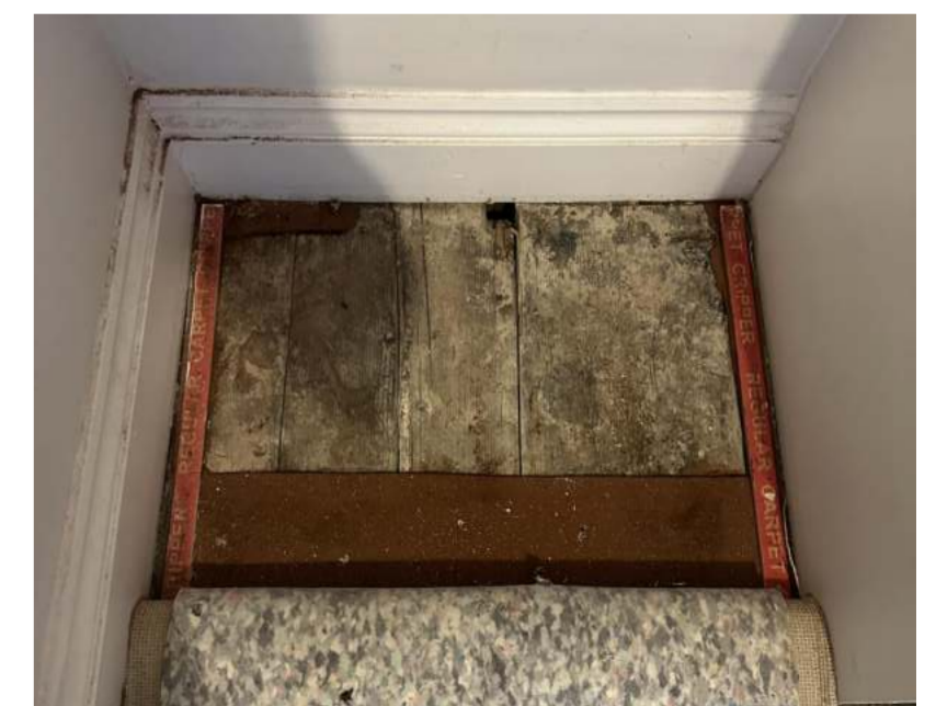
Floor - Photo 2 - Original Floor Boards to be kept
