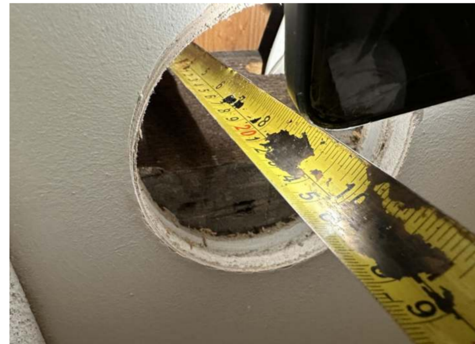
Ceiling - Photo 1 - Plasterboard
