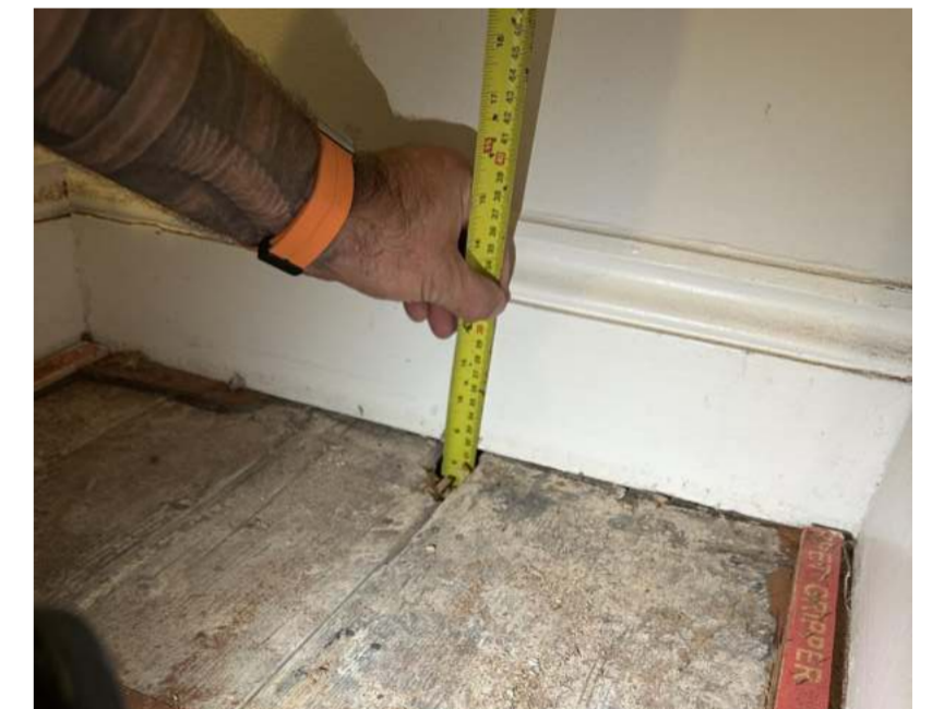
Floor - Photo 1 - Original Floor Boards to be kept
