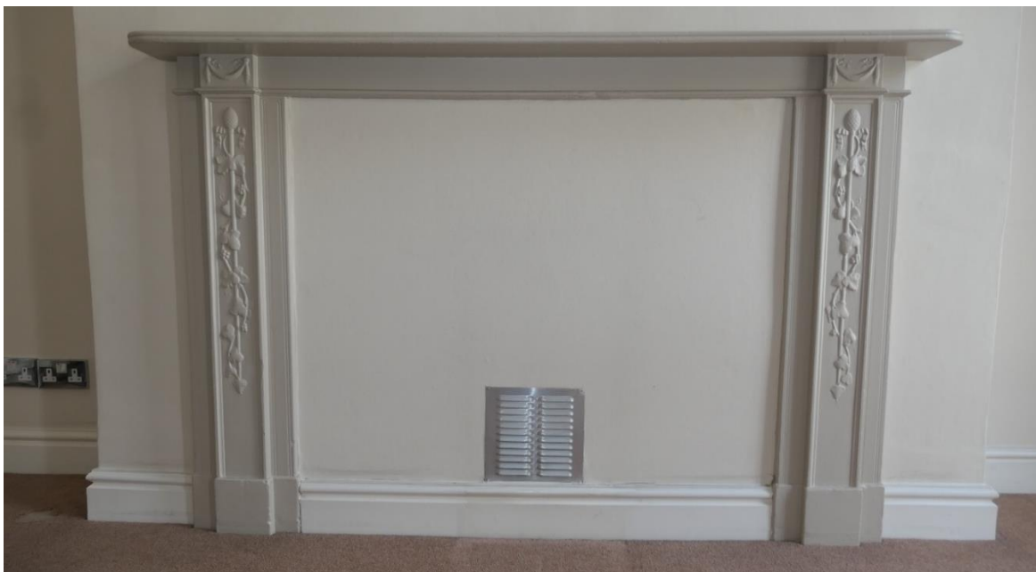
Photo 5: The simple chimneypiece, adorned with a relatively plain Adamesque motif at the front first floor room.
