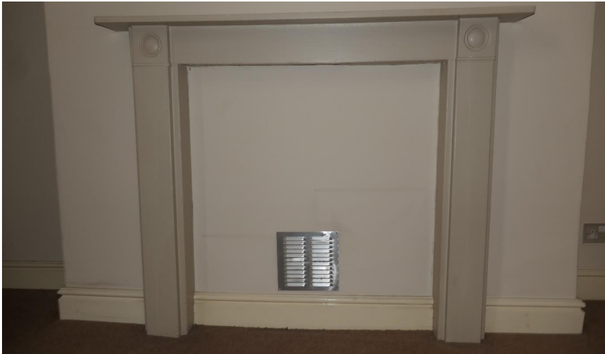
Photo 6: The simpler Regency style chimneypiece to the rear room.
