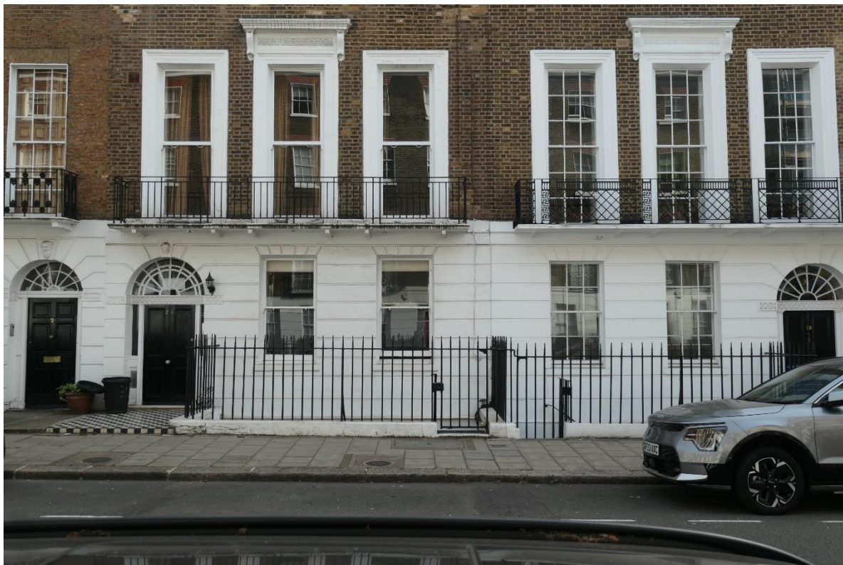
Photo 10: The multi-pane sashes of the buildings adjoining 20 Manchester Street.
