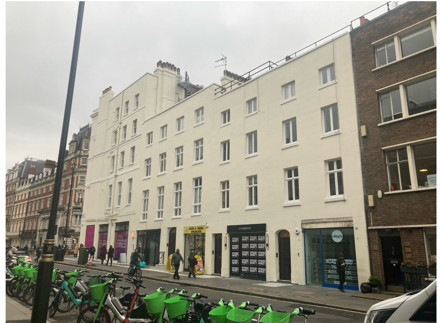
Thayer Street elevation southward
