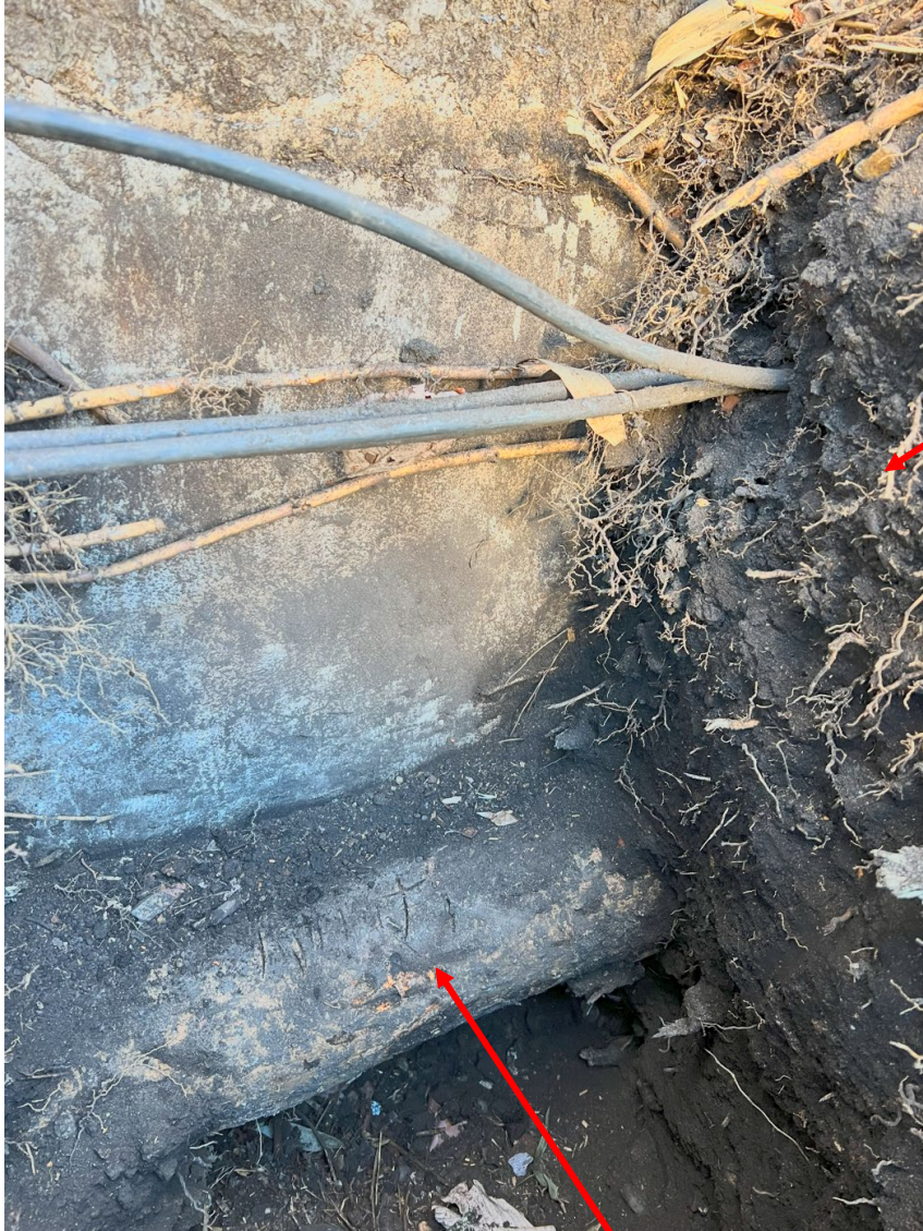
Photograph 1: Trial-pit TP1 – Garden Side
