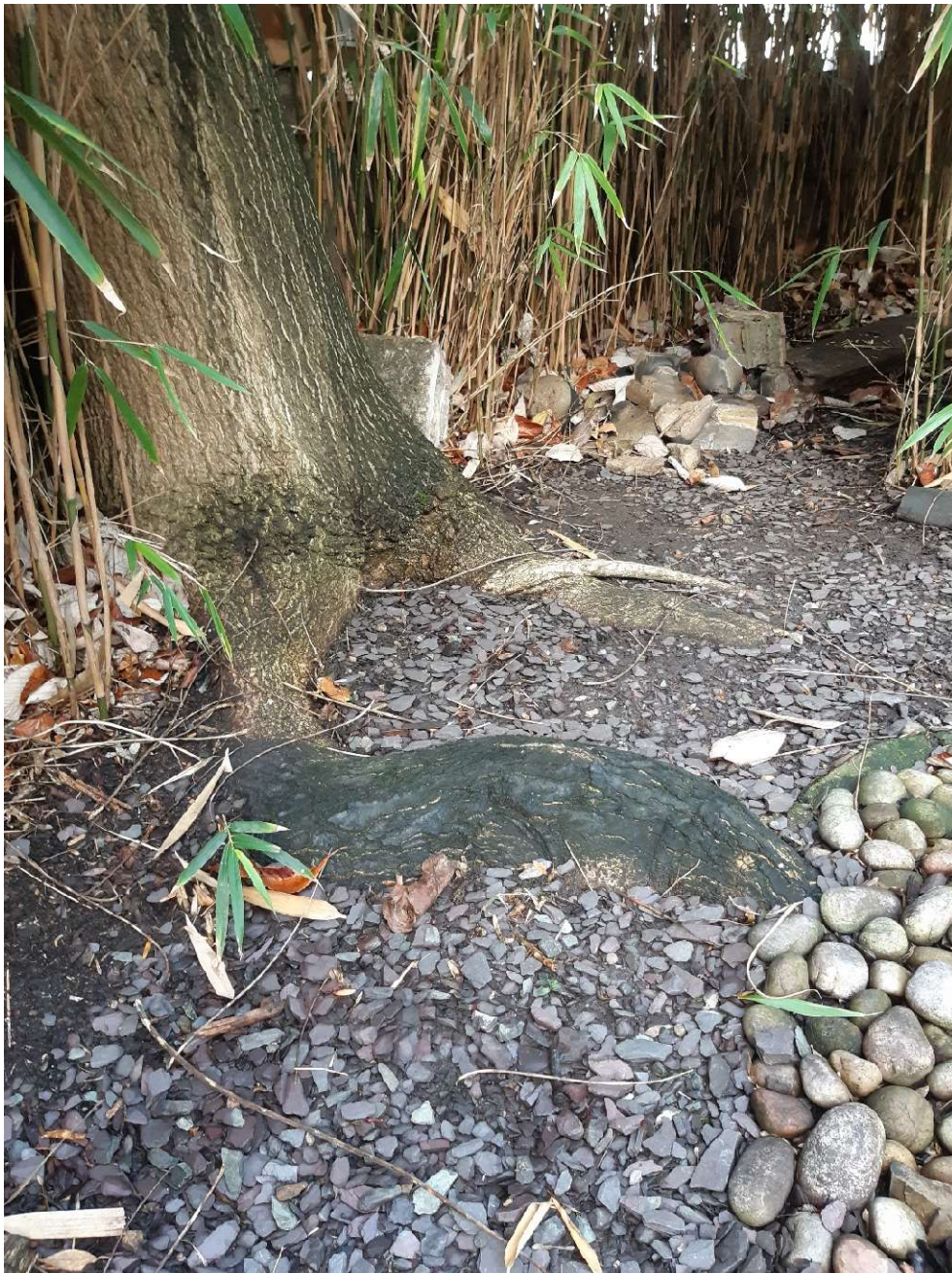
Roots from T1 visible in garden area
