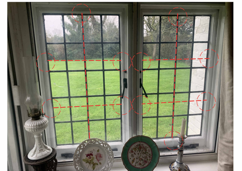
current secondary glazing
