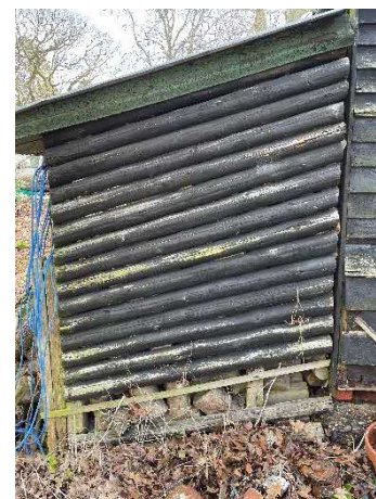
Figure 13 – Lean-to log store to north elevation
