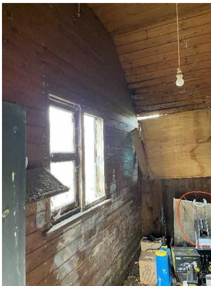
Figure 30 – View of west gable window
