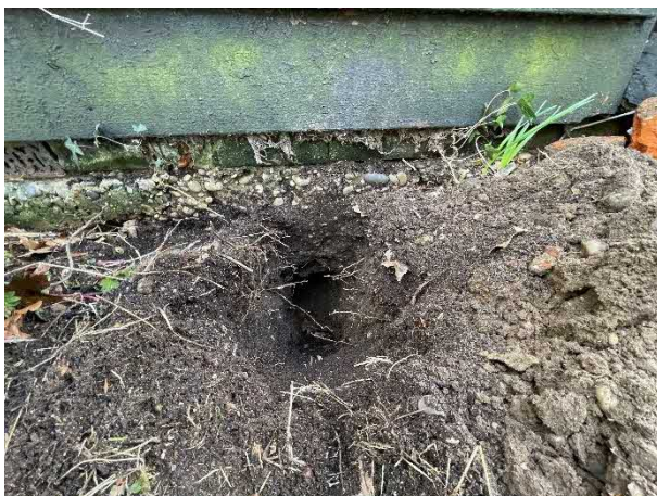
Figure 8 - Trial hole showing concrete floor slab and made ground/soil
