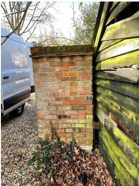
Figure 18 – More modern courtyard brickwork retaining wall adjacent to SE corner
