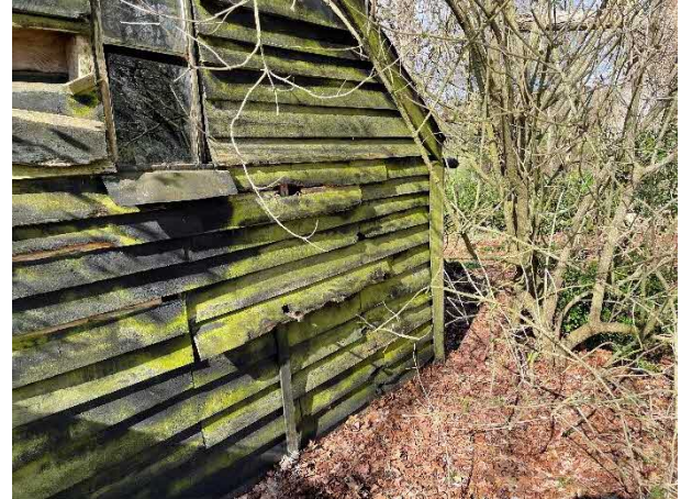
Figure 17 – Lean-to wood store to north elevation
