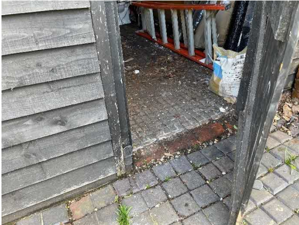
Figure 28 – Third door brick threshold with stable cobble tiles internally and courtyard paving externally
