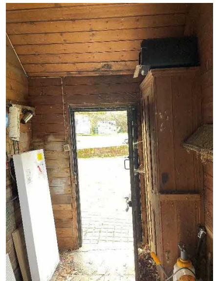
Figure 32 – View to south wall.
