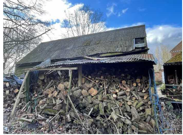
Figure 15 – Lean-to wood store to north elevati
