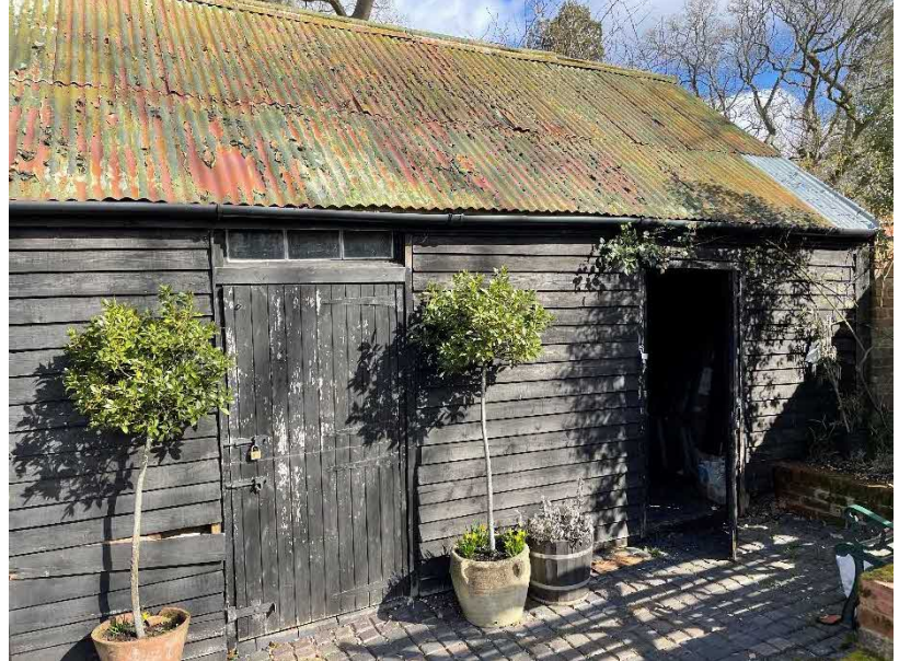
Figure 25 – Lean-to wood store to north elevation
