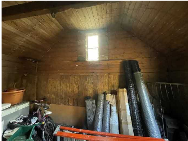
Figure 38 – View of east gable
