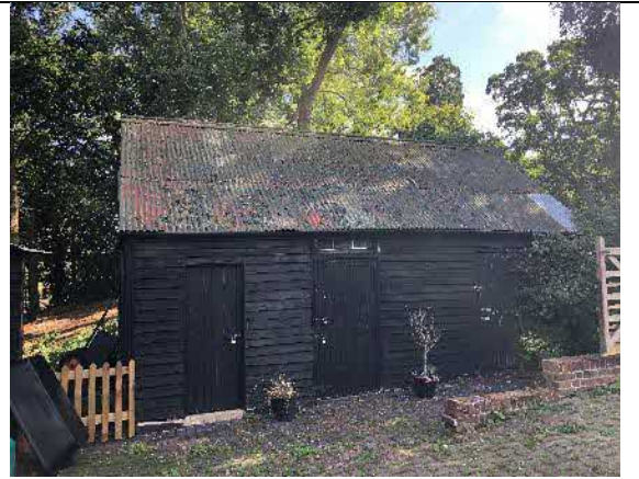
Photograph 2 – Building 2 viewed from the south
