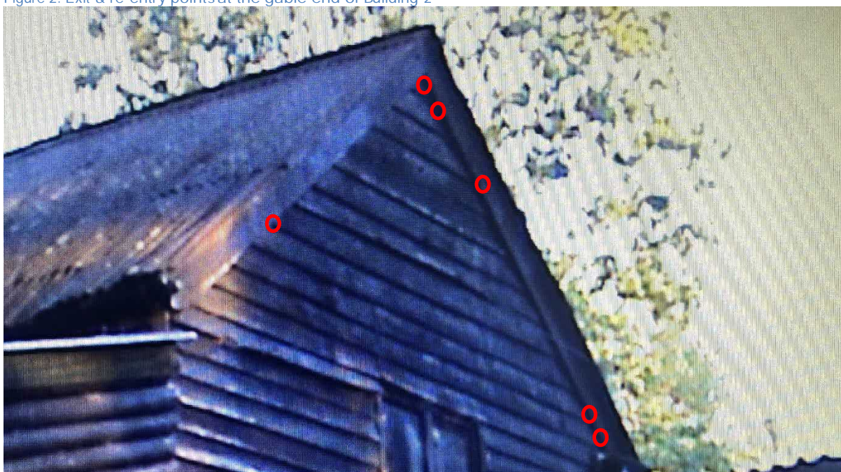
Figure 2. Exit & re-entry points at the gable end of Building 2
