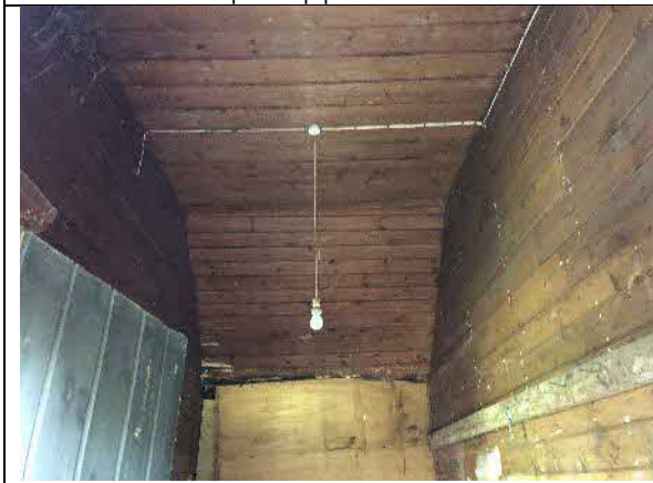
Photograph 3 – Building 2, an internal view
