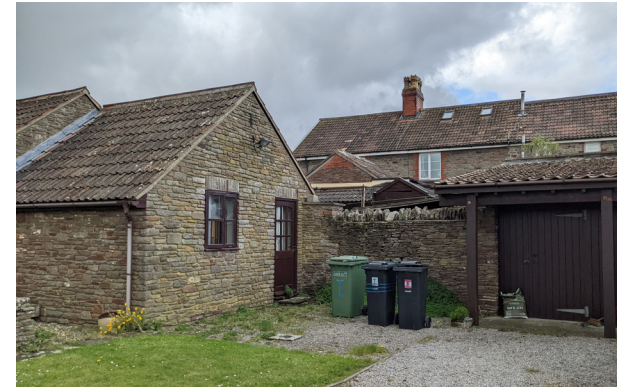
North and east elevation and store / workshop
