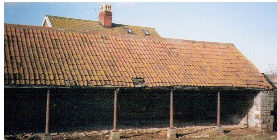
Figure 8 - Ironstones during conversion (the east infill has been removed)
