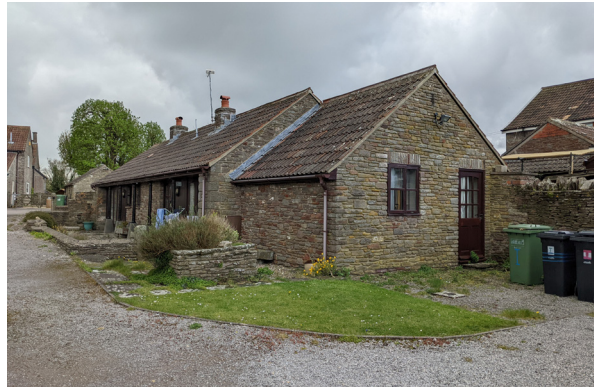
Ironstones, north and east elevation
