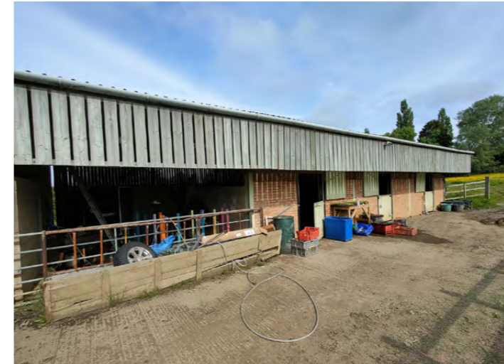
Existing southeast opening and stable doors
