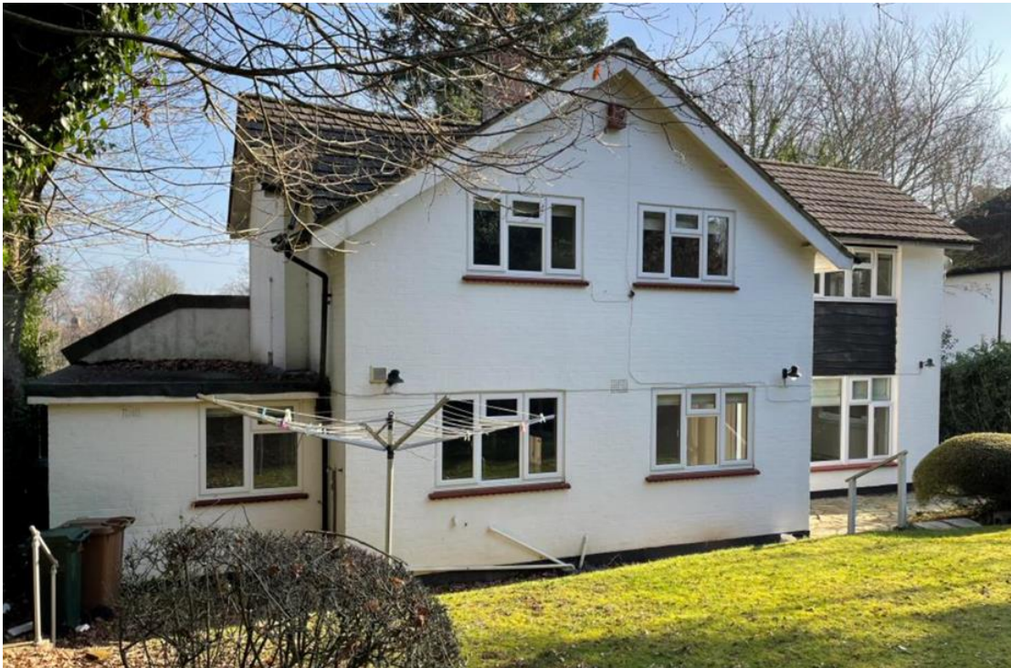
Fig.3: Rear elevation with garage to left.
