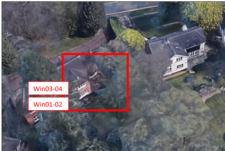
Figure 3 – Neighbouring Windows at No 2 North Approach (numbering is from left to right)
