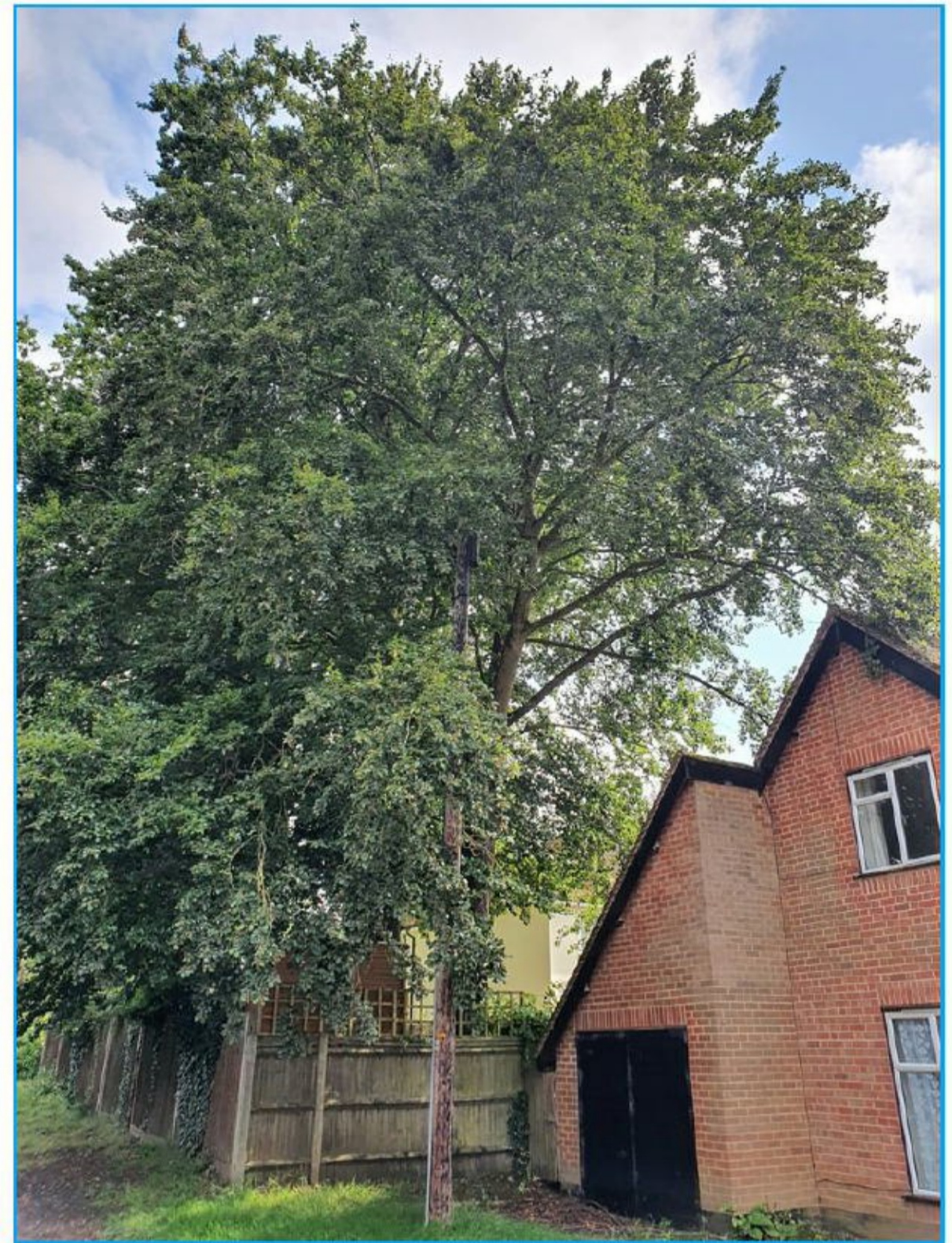
Fig 2: Small extension under tree #01- for demolition
