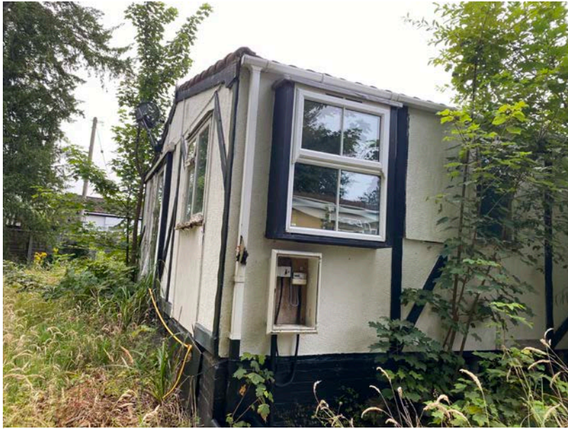
North-western elevation of B1
