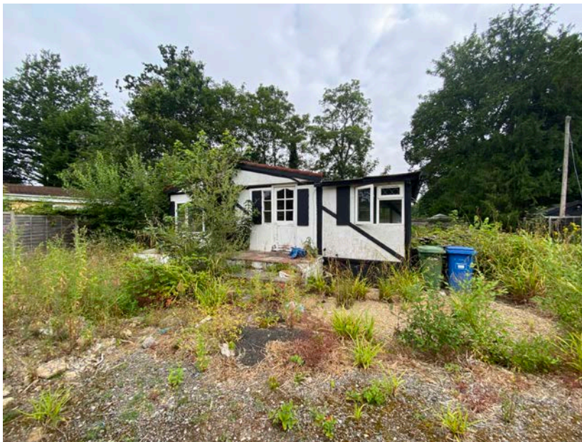
Southern elevation of B1
