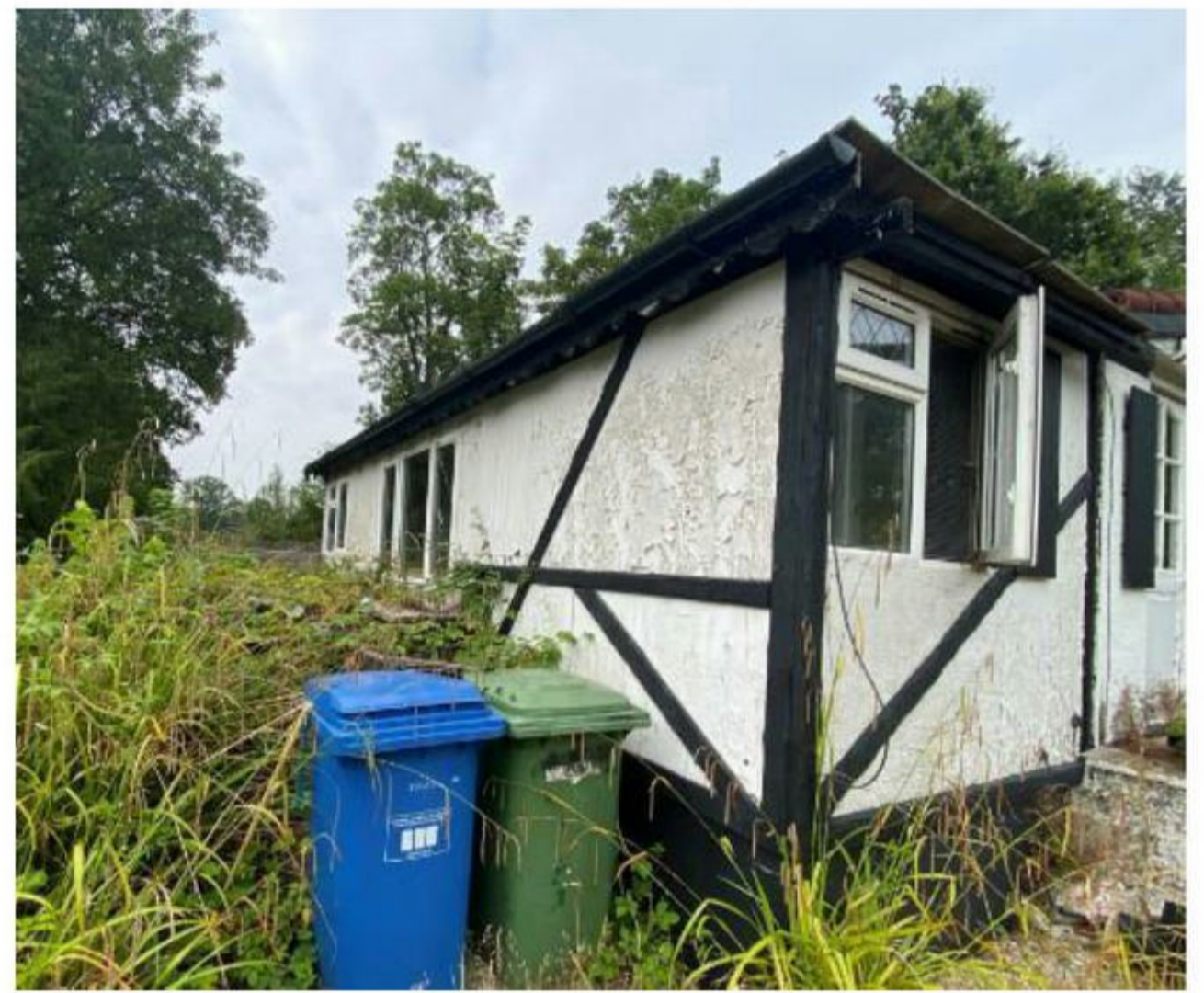
Photo 4: South-western elevation of B1
