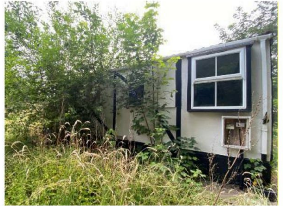
Photo 2: Western elevation of B1
