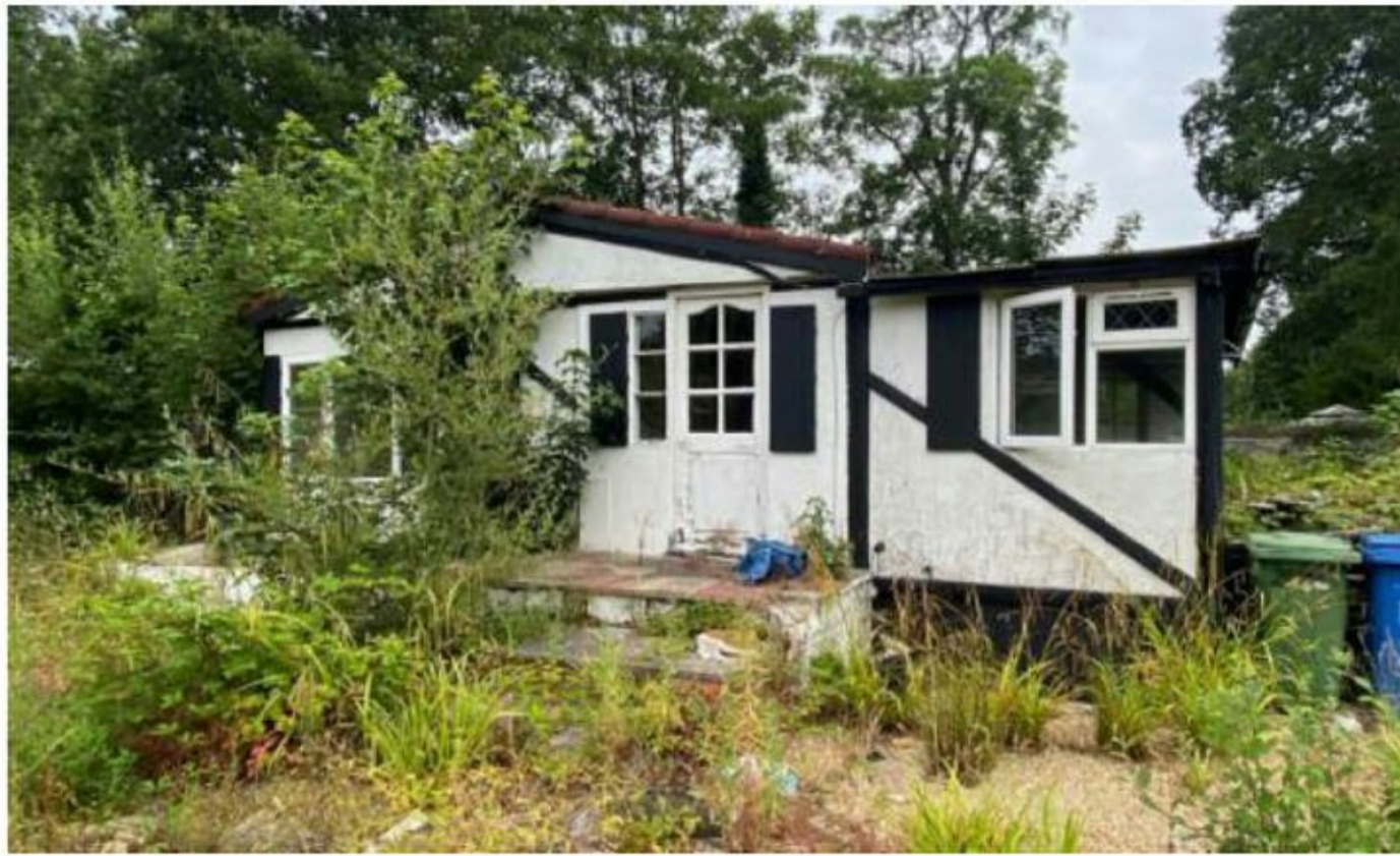
Photo 1 : Southern elevation of B1
