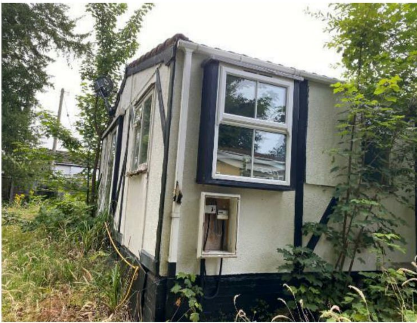
Photo 3: North-western elevation of B1
