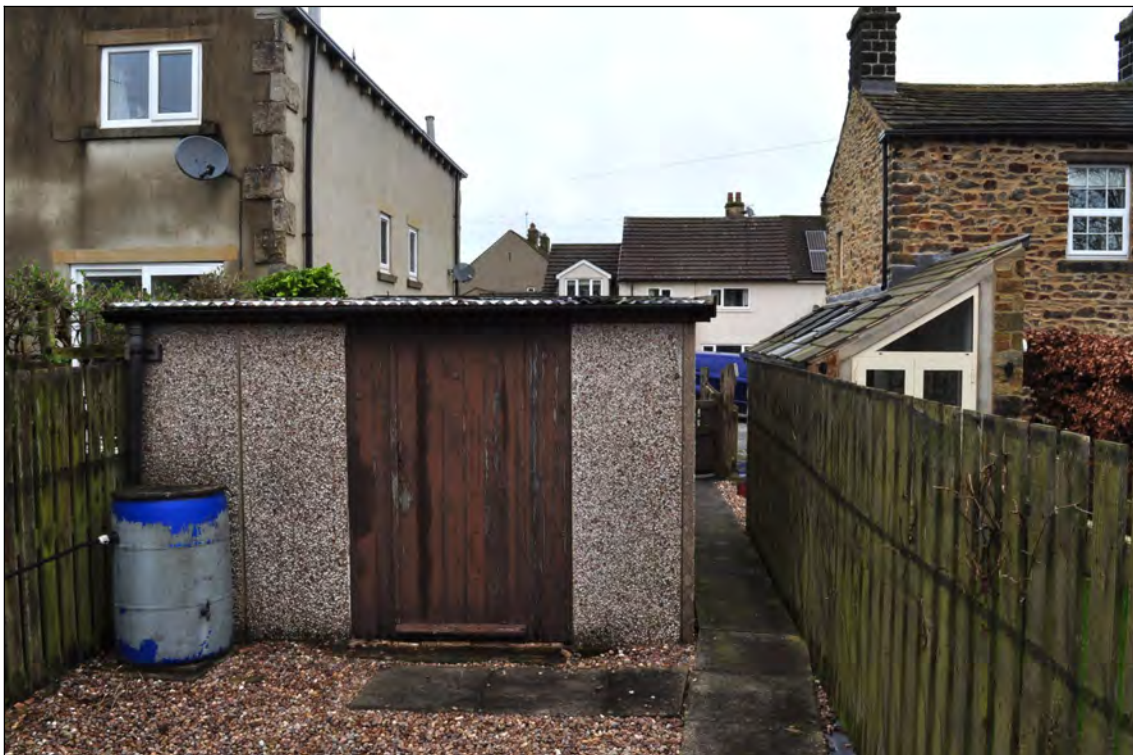
Photo 2: Existing garage within application site, looking north
