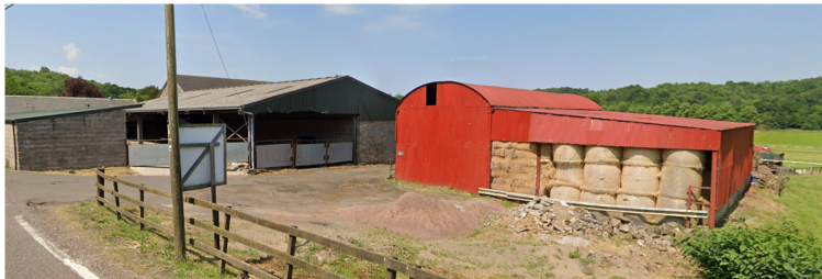
Photograph of nearby agricultural buildings featuring metal cladding and roofing.
